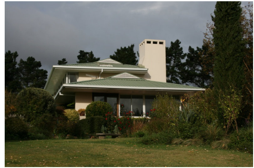
3. View from the garden looking east
