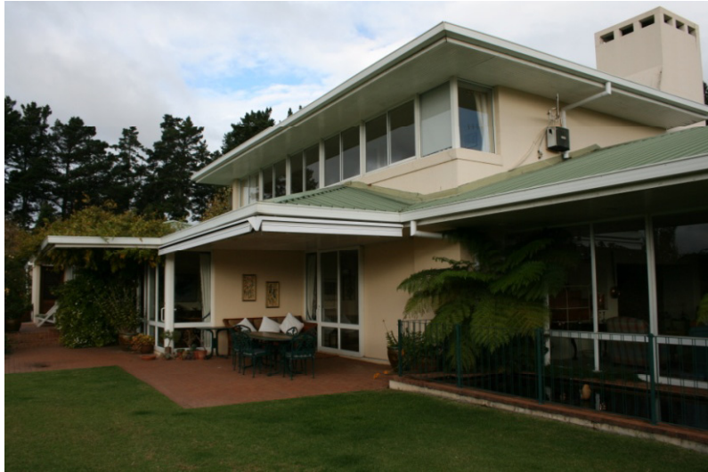
4. View from the garden looking south-east
