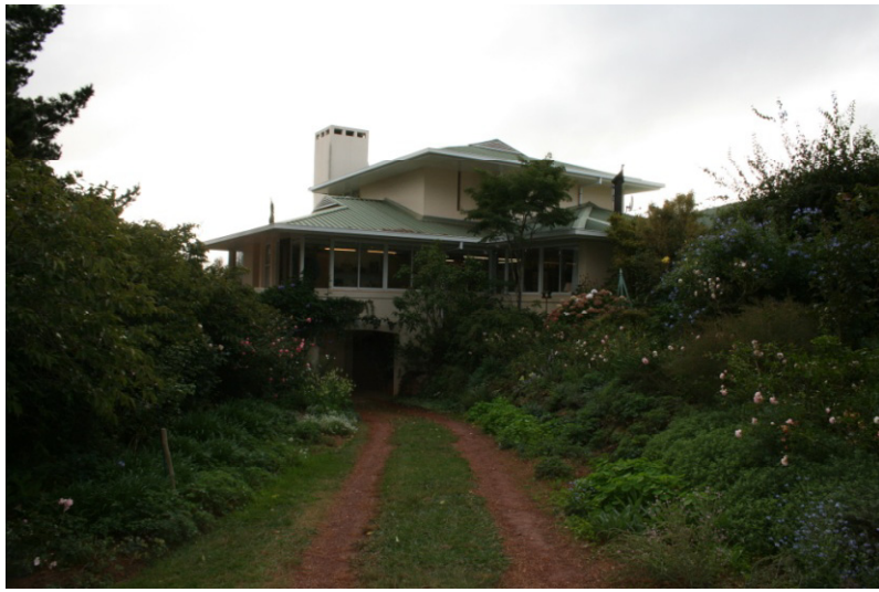
1. View from the driveway looking north-west
