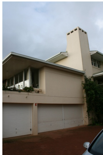
8. View of the south-west corner
