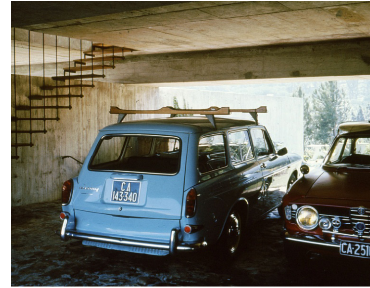
3. View looking north showing suspended stairs
