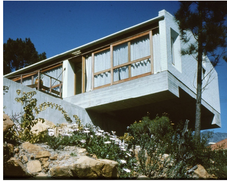
2. View from the garden looking south showing cantilever
