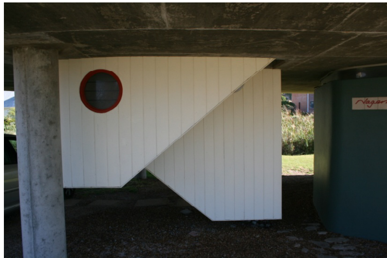
4. View looking north-west showing suspended stairs
