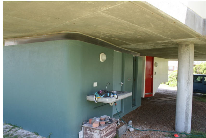
5. View looking south showing storeroom
