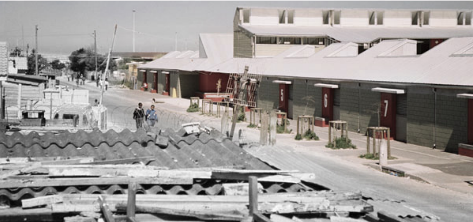
Fig 5.11_ Usasazo Secondary School, view from the street, showing temporary entrepreneurial teaching classrooms
