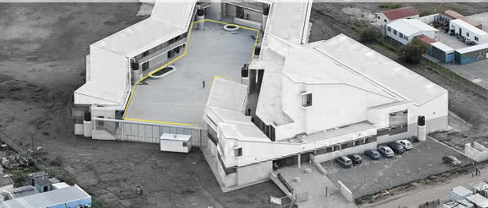
Fig 5.17_ Inkwenkwezi Secondary School, aerial view of introverted courtyard and building mass
