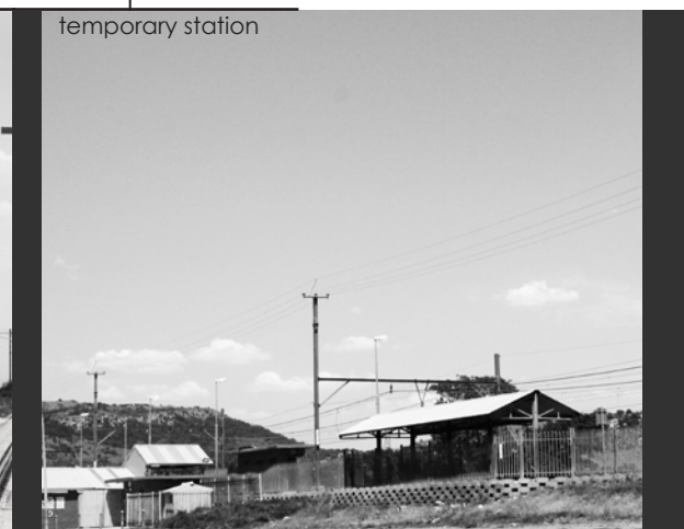
Figure 03-5 Pienaarspoort Station, by author (March 2012)
