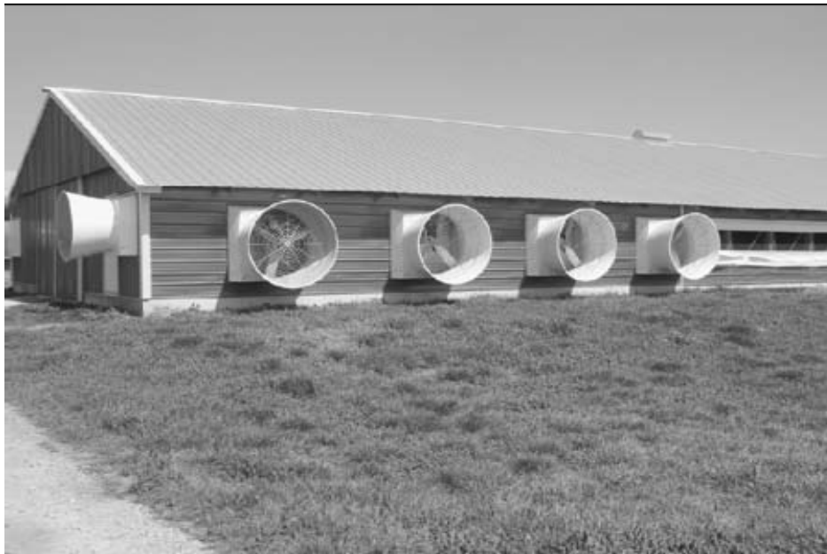
Fig. 2.3. Fans located at one end of a poultry house, to allow for cooling by with wind chill and/or evaporative cooling (For this specific house, the air was cooled by a water drive heat exchange system)(Source: Czarick and Fairchild, 2008).
