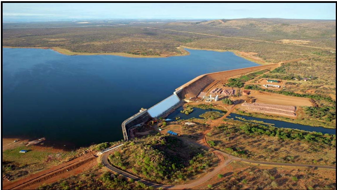
Figure 7: The Flag Boshielo Dam with outflow into the Olifants River and construction site visible across the Olifants River.
