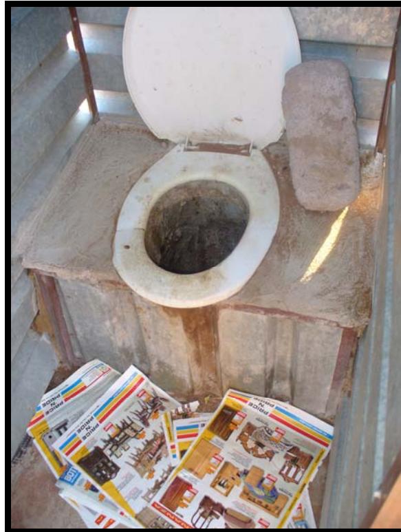
Figure 4.5: A typical pit toilet used in both study villages in the Vhembe region of the Limpopo Province, South Africa: no toilet paper available and people used old magazines and newspapers
