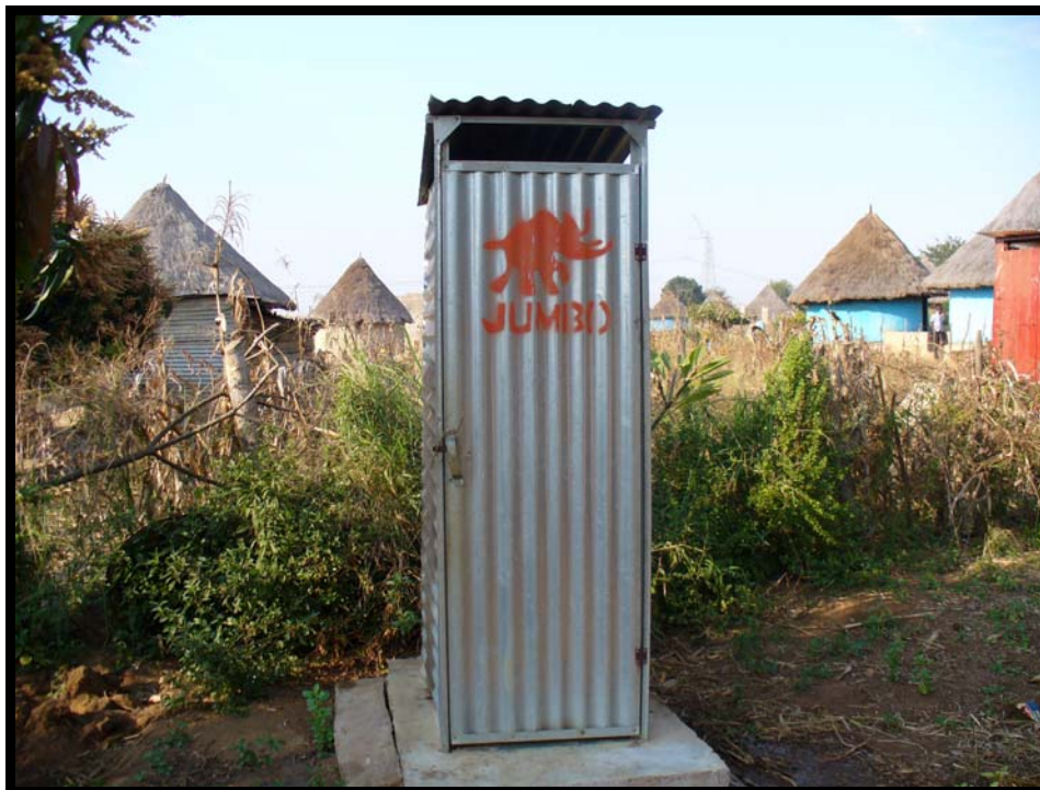
Figure 4.6: A VIP toilet used in both study villages in the Vhembe region of the Limpopo Province, South Africa
