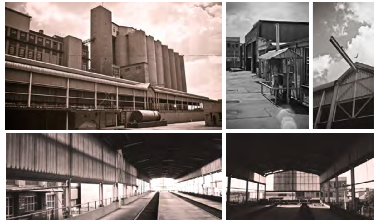
_2.5 Photographic study of the structures and spaces on the site.
