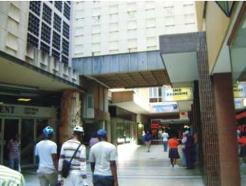
FIGURE 3.41 View showing pattern of open and covered areas
