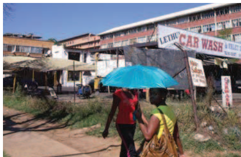
illus. 6.5 Sidewalk in need of upgrading and vegetation overgrowing fence
