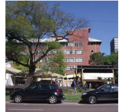
illus. 4.22a A.J.O. Centre. Eastern facade from site
