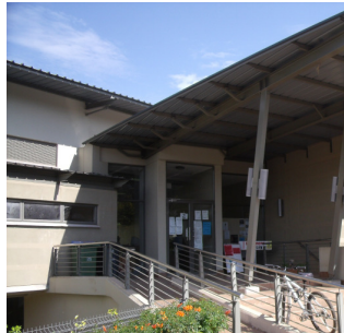
illus. 3.3b Alkantrant Library Ramp 1, stair 1
