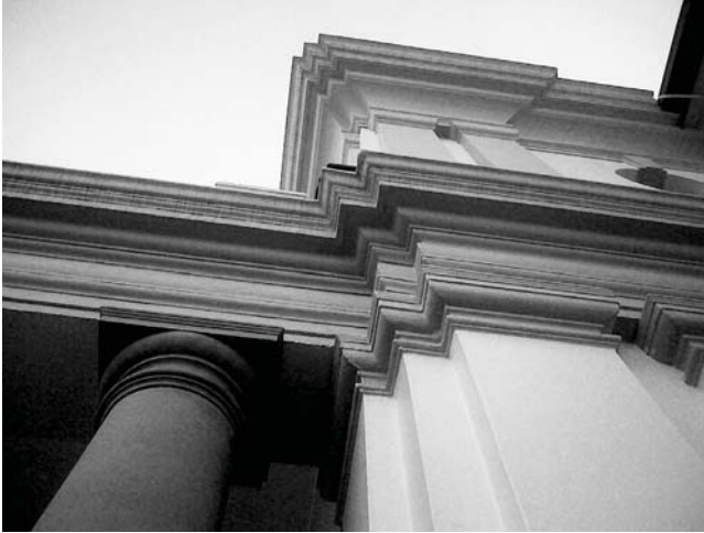
Illustration 5.4 Exterior wall of The Tshwane District Hospital
