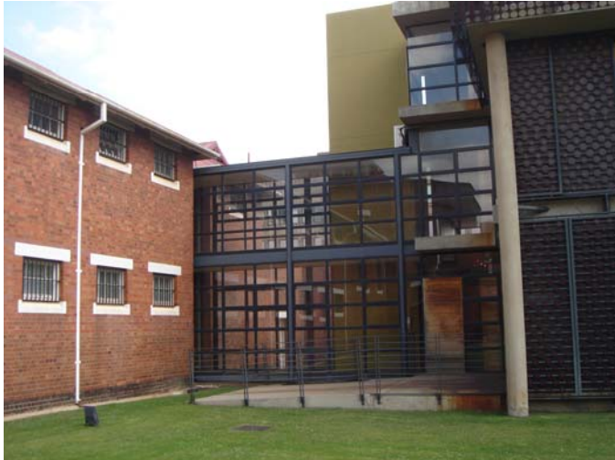
Fig. 6.8: New Architecture juxtaposed to the Existing Building
