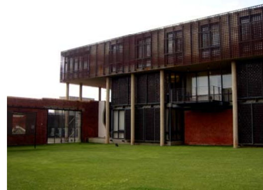
Fig. 6.7: View from Courtyard to the East Wing
