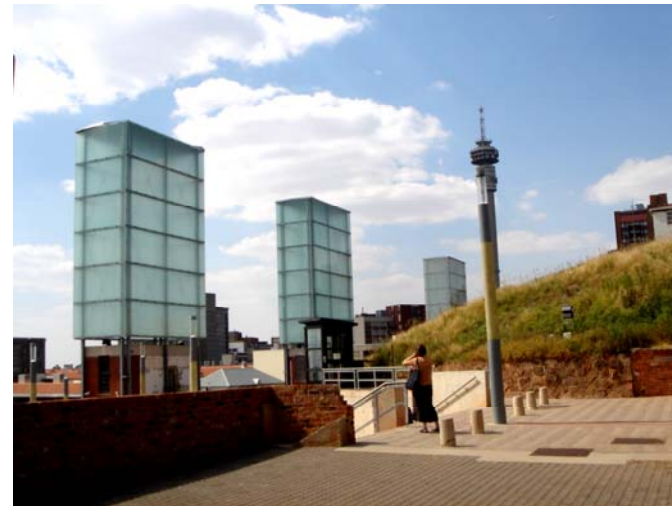
Fig. 5.14: View of the Awaiting Trial Block Stair towers in the Public Square at the Constitutional Court
