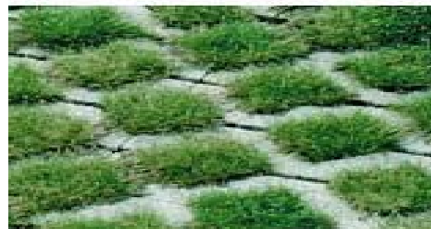
Fig. 8.7: Grassed Pavers and Permeable Concrete
