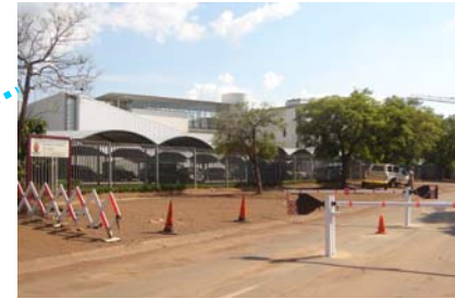
Fig 3.7(a): View of north boundary of the site
