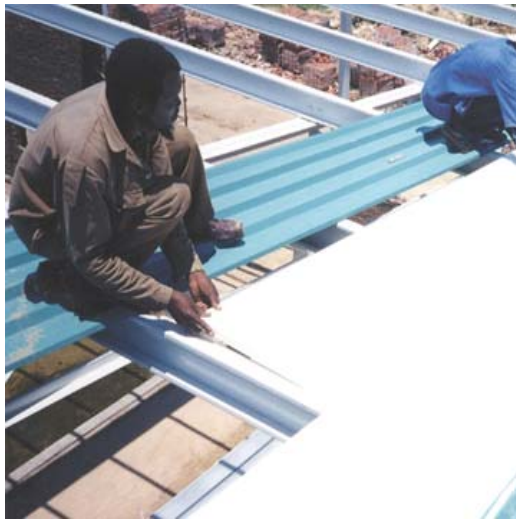
Fig 8.6: IsoBoard Insulation
