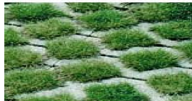
Fig. 8.7: Grassed Pavers and Permeable Concrete
