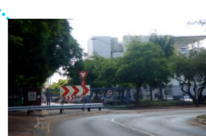
Fig 3.7(c): View of the Duxbury Street entrance which is intended to be reopened by the University
