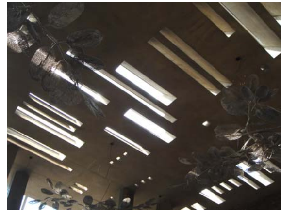
Fig 5.10: The ceiling of the foyer in the Constitutional Court. The skylights seek to recreate the dappled light under a tree.
