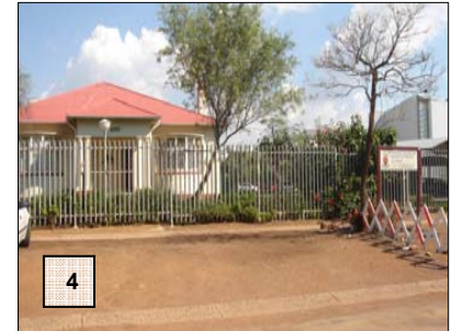
4 House used as Catering Offices
