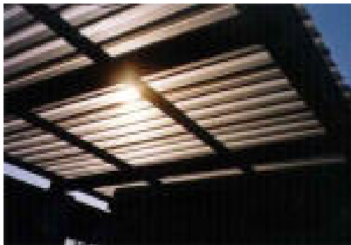
Fig 8.9: Polycarbonate translucent roof sheeting
