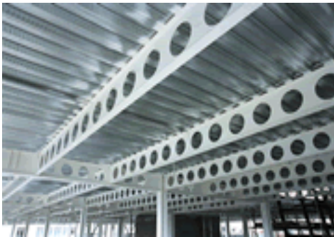
Fig 8.2: Macsteel Cellular Beams
