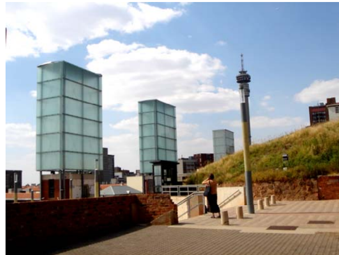
Fig. 5.14: View of the Awaiting Trial Block Stair towers in the Public Square at the Constitutional Court
