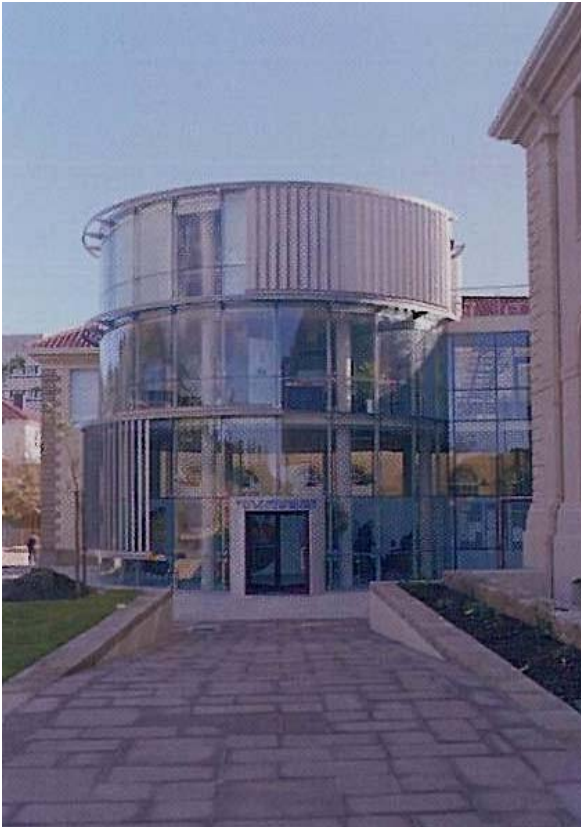
Fig. 6.2: Entrance to the Link Building
