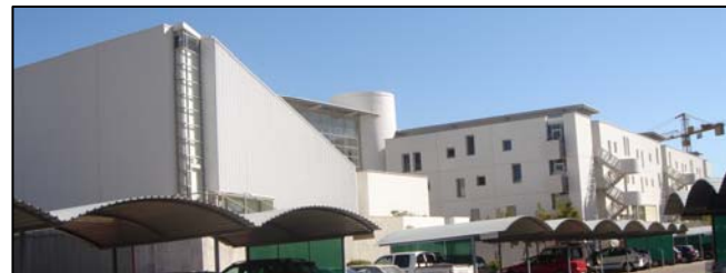
Fig. 3.13: The North Façade is more solid than the south with sheer white carefully punctured walls
