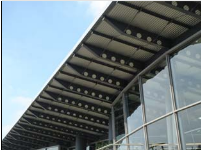
Cellular beams at Audi Car Sales Centre, Corlett Drive, Johannesburg
