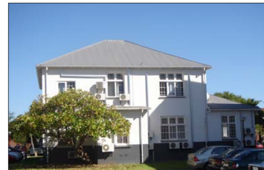
Fig. 3.9: Rissik House (photographs by author, March 2008)
