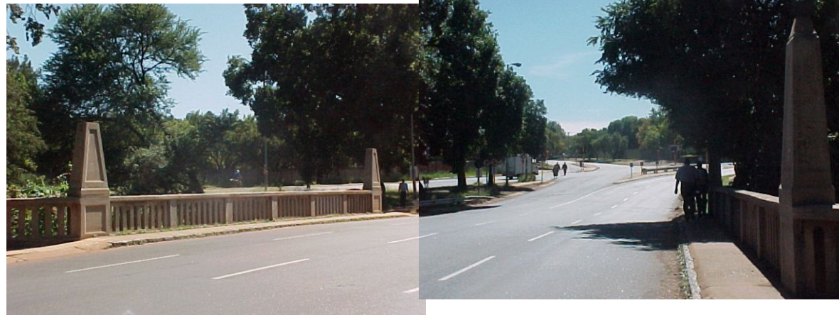
2.43 Bain and Proudfoot's 1932 bridge across the Apies River with Dr Savage street across it
