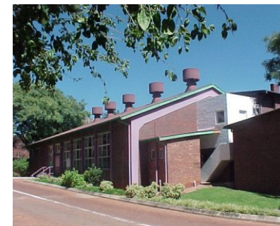
2.40 Older industrial buildings
