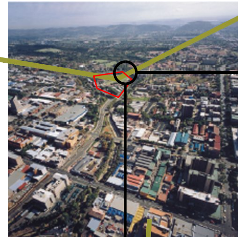
2.12 Site overview from the south
