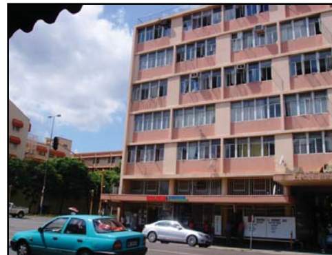
fig.6.9. Lion Bridge Building (classrooms and staff accommodation)
