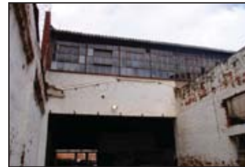
fig.2.11. Industrial / Automotive building types in precinct
