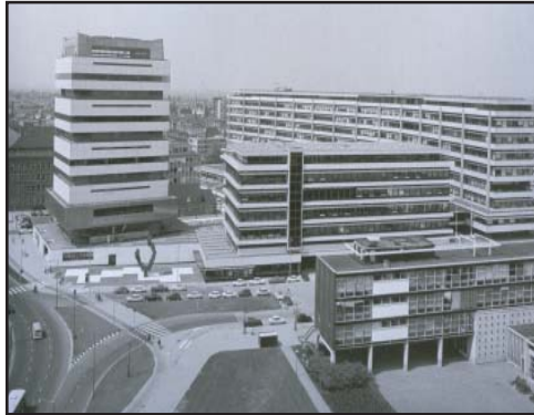
fig.7.17. Aerial view of the Akragon and Technikon
