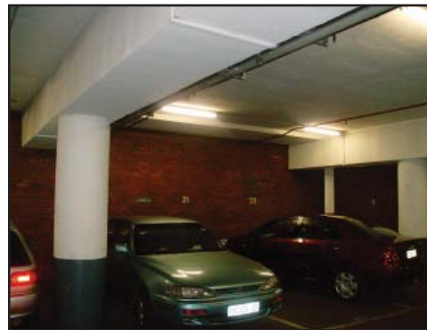
fig.5.23. Parking bays located in-between existing columns
