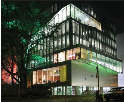
fig.7.25. Different lighting techniques and glazing colors reinforce the architectural intentions
