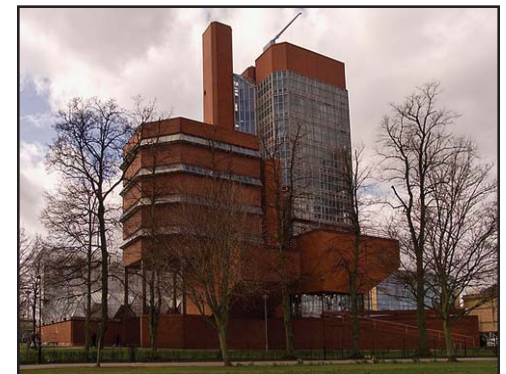
fig.7.24. View from campus showing 45 degree angled glazing protruding from heavy brickwork on secondary tower
