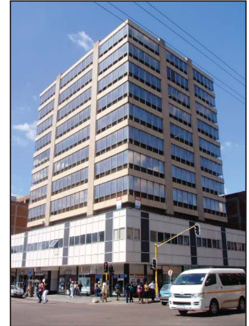
fig.5.2. The Apollo Centre on the corner of Church and Du Toit Street
