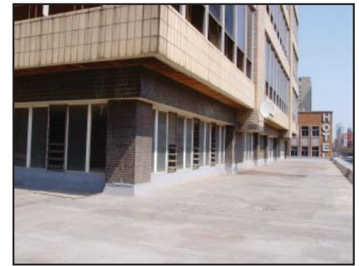
fig.5.35. Exterior second floor area (first floor rooftop)
