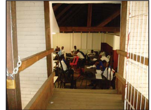
fig.6.13. Drywall partitioning used to create classroom spaces
