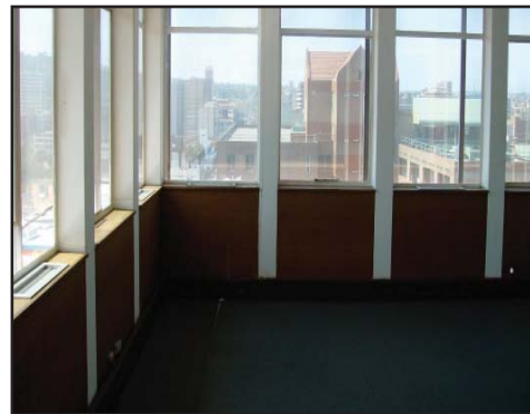
fig.5.38. Concrete columns periphery
