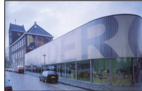
fig.7.33. Bredero School Building
