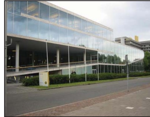
fig.7.20. The structural form expresses and complements its function
