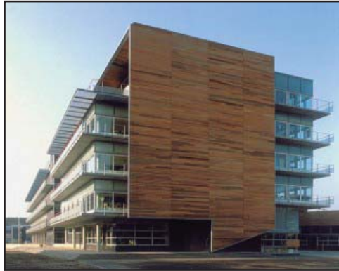
fig.7.29. A Timber clad skin conceals the main circulation volume
