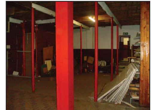
fig.6.14. Steel supports inserted for wooden flooring above
