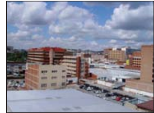
fig.2.10. Industrial / Automotive building types in precinct
