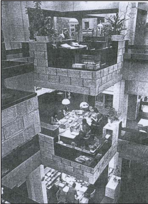
fig.7.8. Personalized working platforms cantilevering into the central atrium
