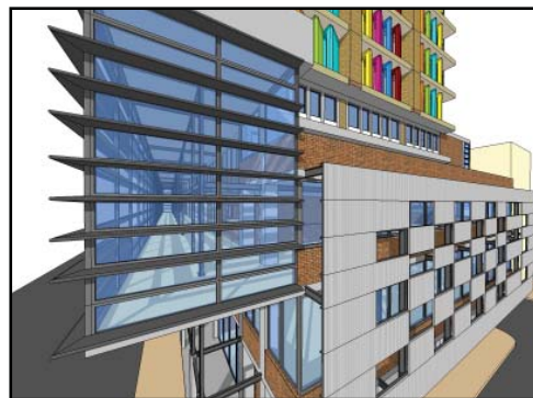
fig.10.27. Glazed facade wraps around to western side with the corrugated western screening continuing on the western facade
