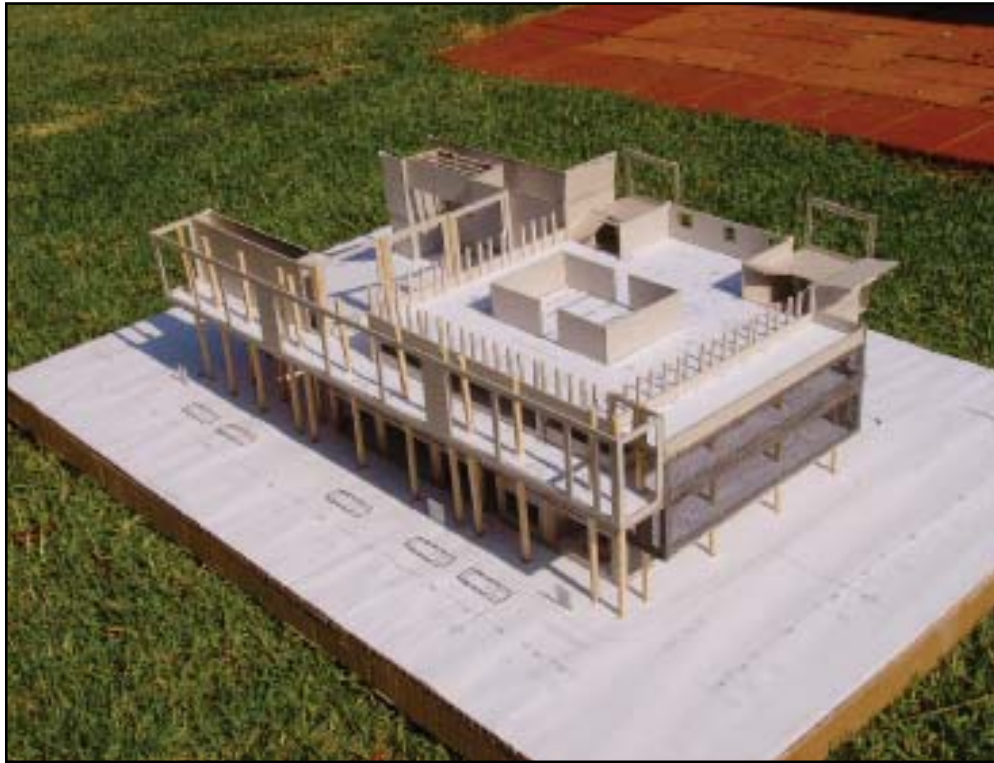
fig.9.152. Bird's eye view of model showing structural composition of first three floors of the proposed altered structure
