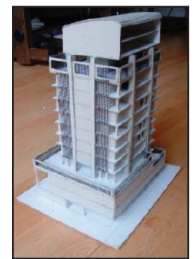
fig.9.19. Model showing multi-purpose rooftop hall as well as the use of vertical screens on the eastern and western facades
