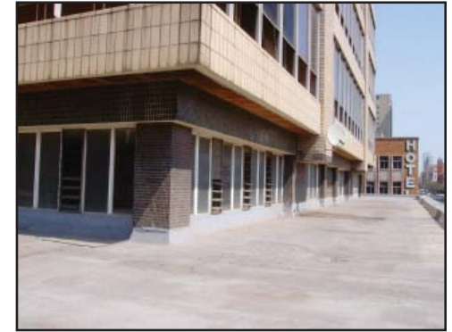
fig.5.35. Exterior second floor area (first floor rooftop)
