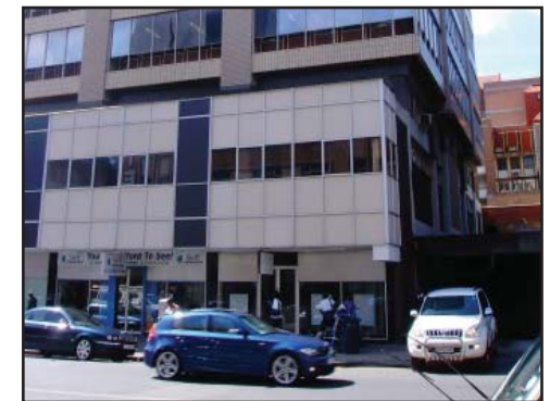
fig.5.19. Vehicular entrance to the Apollo Centre from Du Toit Street
