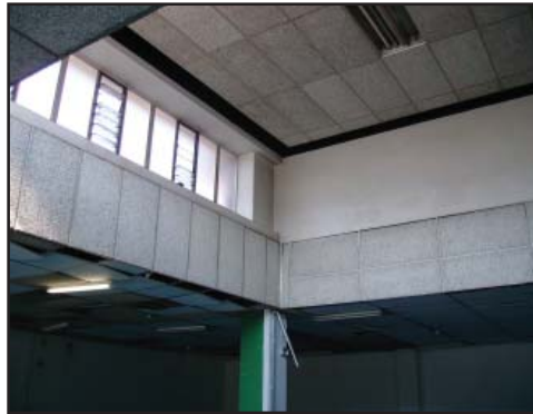
fig.5.33. Double volume spaces that are connected to the first floor
