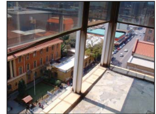
fig.5.40. Tinted, glazed sunscreen panels fixed to concrete overhangs
