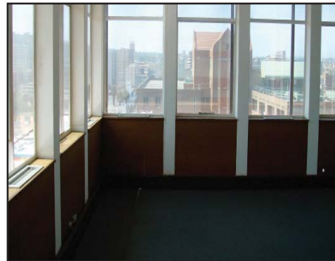
fig.5.38. Concrete columns periphery
