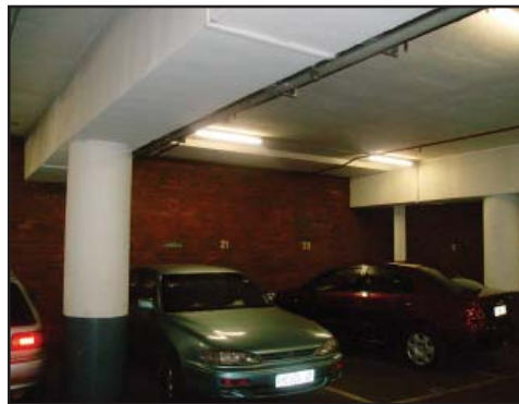
fig.5.23. Parking bays located in-between existing columns
