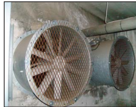
fig.5.24. Mechanically ventilated basement cavity walls
