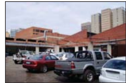
fig.2.12. Industrial / Automotive building types in precinct
