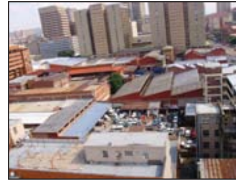
fig.2.9. Industrial / Automotive building types in precinct
