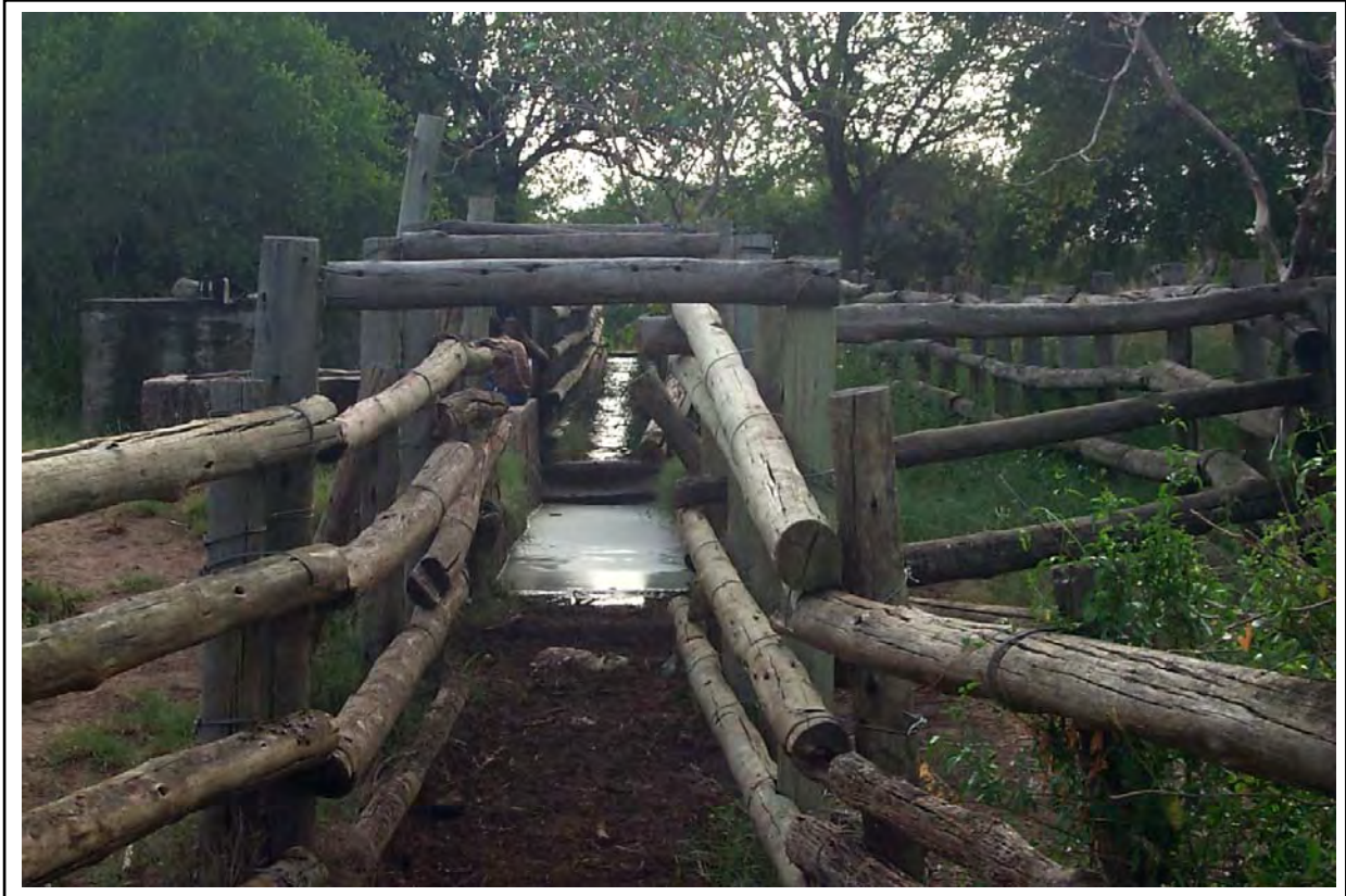
Figure 3.8: The Nhlanjwana concrete dipping tank at Mbangweni in Maputaland, KwaZulu-Natal.
