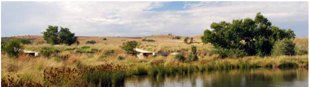
Figure 4.10 View over the planted sod roofs
