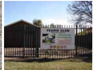
Figure 3.17 Faerie Glen sub-station
