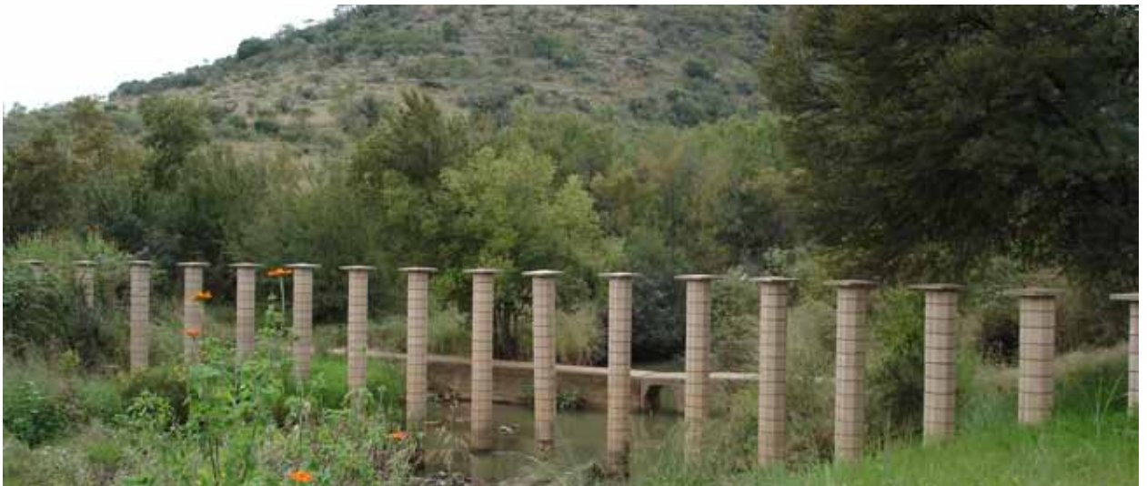
Figure 3.69 Stormwater debris trap with pedestrian bridge behind it
