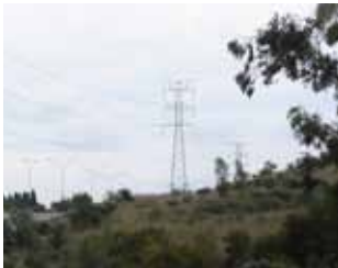
Figure 3.14 High voltage powerlines
