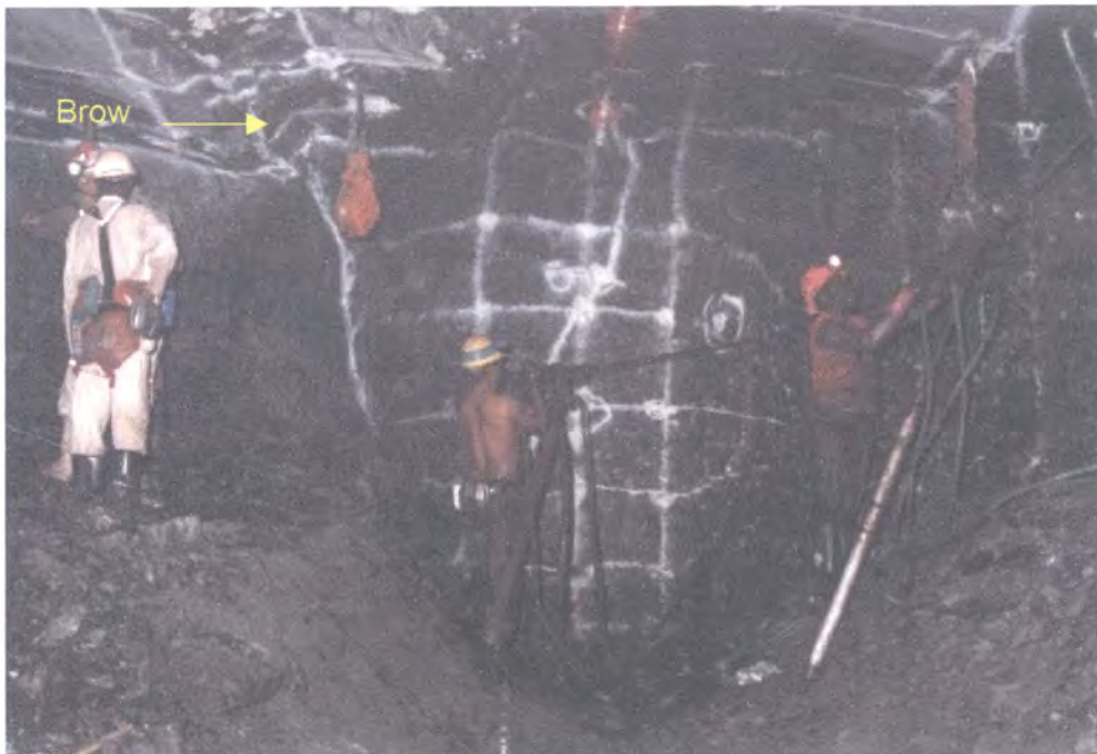
Figure 4.43 – Development-type round with a burn cut, used to advance an ASG-type gully, here shown in a high stope width area at shallow depth
