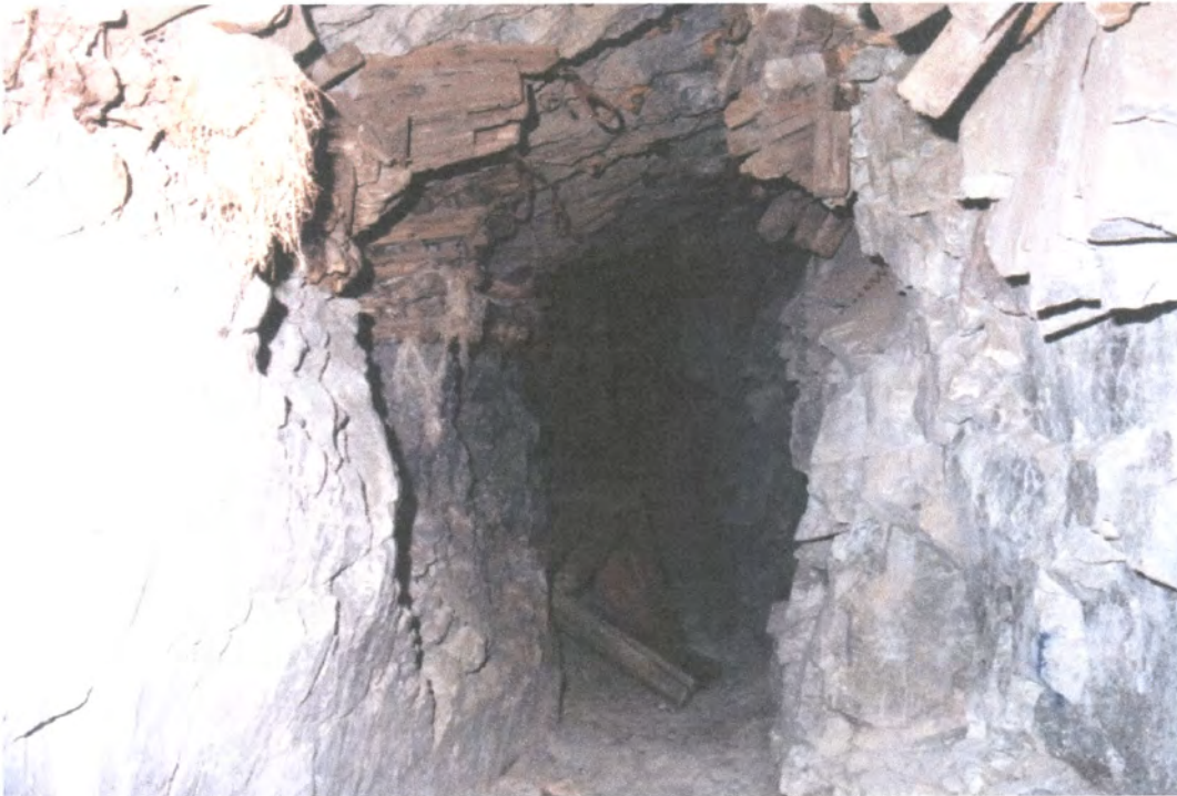
Figure 4.47 - VCR – good blasting practice - footwall lifted gully advanced incrementally by drilling horizontally in the gully face
