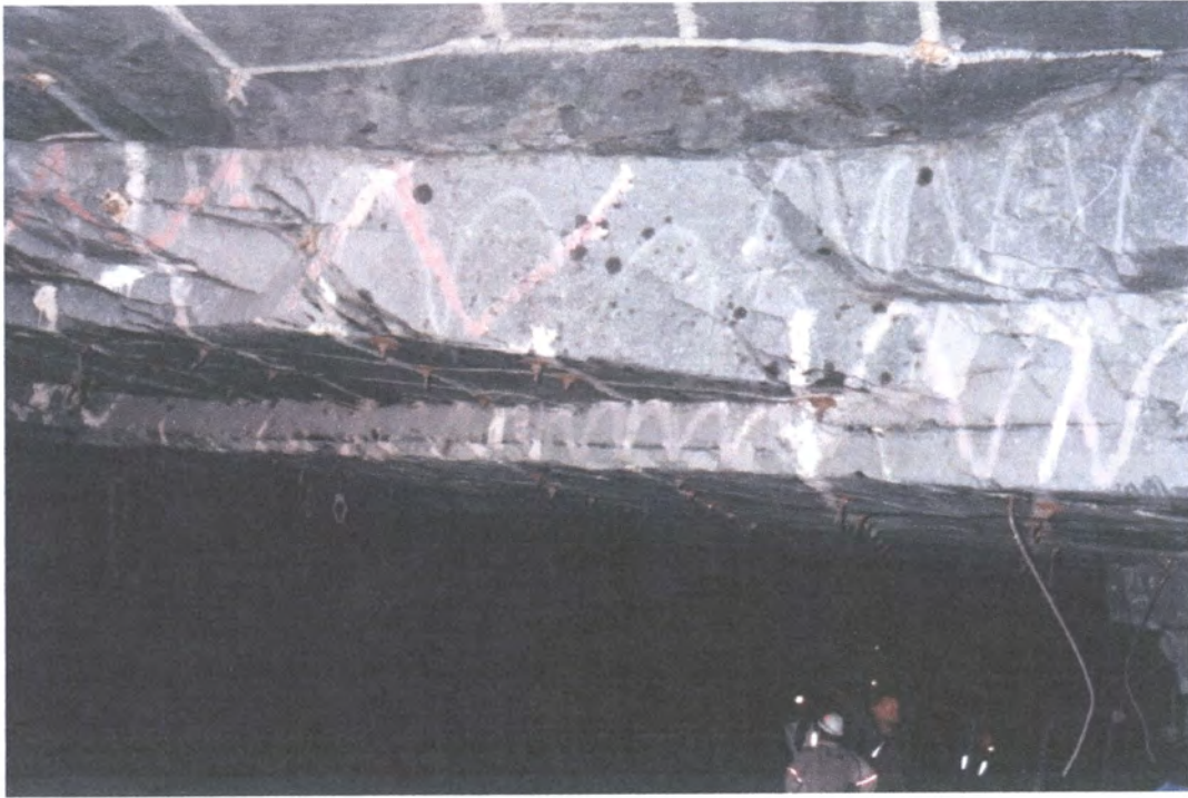
Figure 4.11 - Brow in massive, bedded quartzite over a gully on the Beatrix reef at 900 m depth
