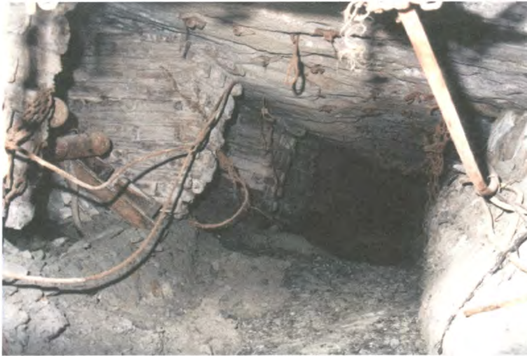
Figure 4. 35 - VCR footwall lifted gully – good hangingwall conditions
