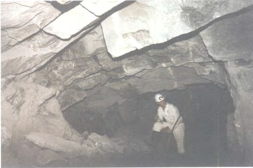
Figure 4.13 - Zone of dense jointing creating a hazard on the Merensky Reef at 600 m depth. Siding left on left side of gully and additional in-stope pillar left on right
