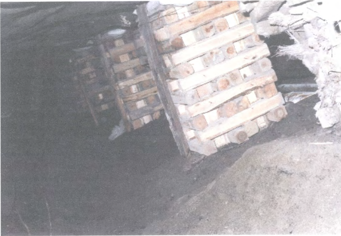
Figure 4.49 – Correctly constructed packs, normal to reef, prestressed, with a grout bag
