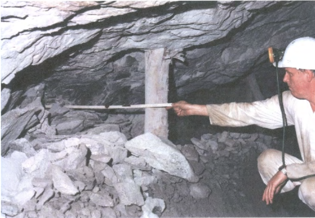
Figure 4.17 – Merensky Reef - lagging 1 m wide supported siding
