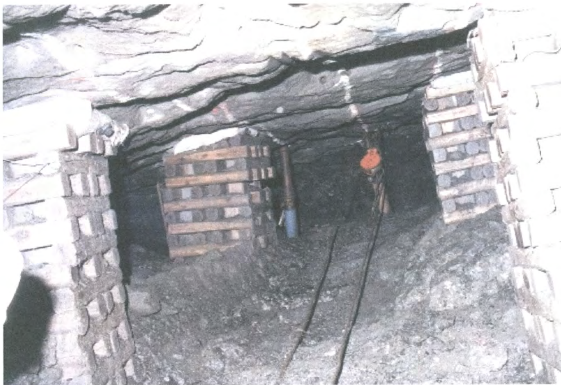
Figure 4.23 - Merensky Reef - conditions in a wide heading with footwall lifted gully
