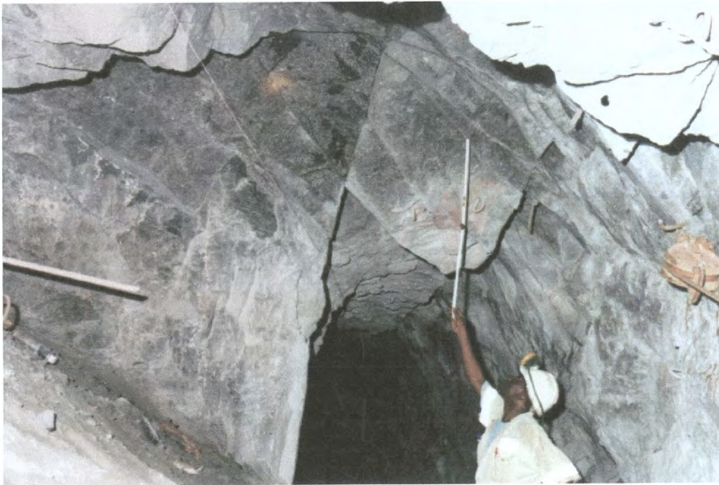
Figure 4.12 - Hazard resulting from joint-bound wedges over a strike gully on the Merensky Reef at approximately 300 m depth. An additional pillar is left on the up dip (left) side of the gully to reduce the risk of a fall
