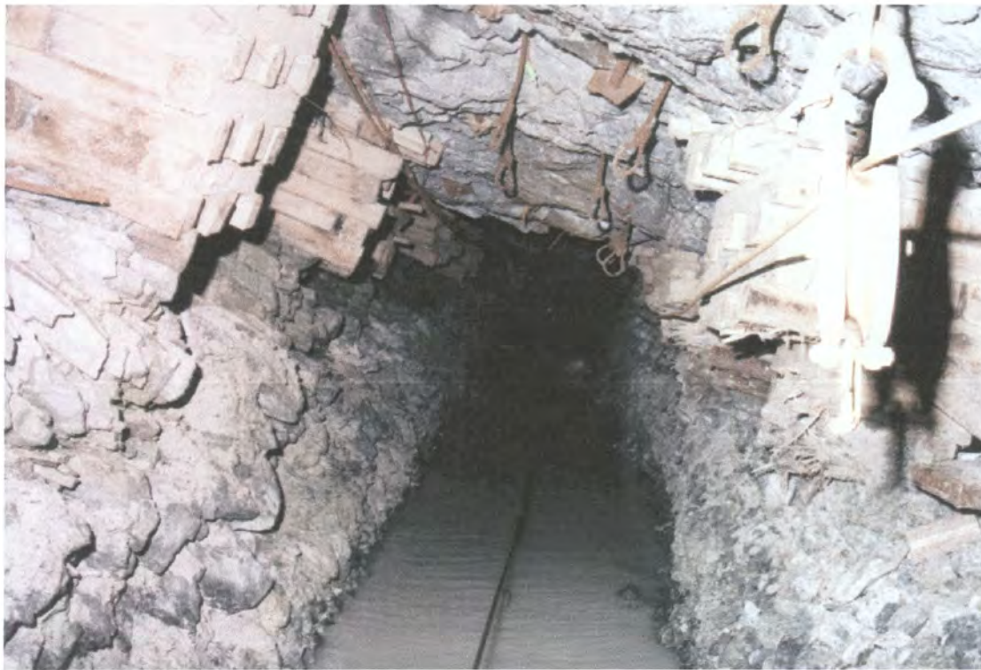
Figure 4.34 - Carbon Leader wide heading footwall lifted gully with good hangingwall conditions at 3200 m depth
