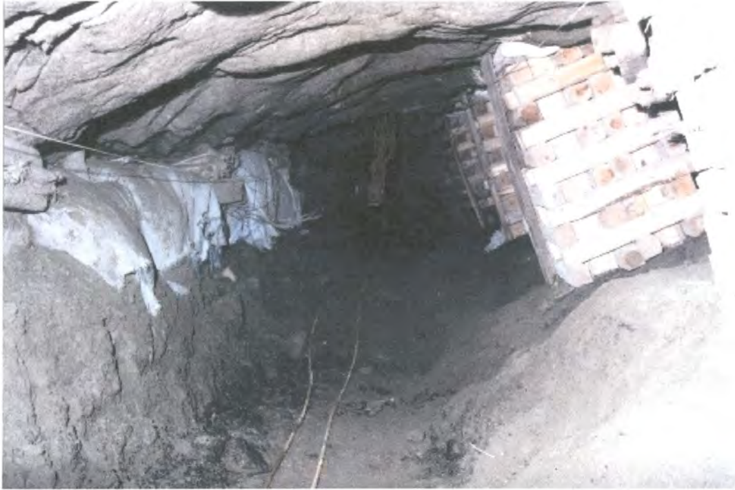
Figure 4.24 – Conditions along a footwall lifted gully on the Merensky Reef. Note backfill installed on the down dip side
