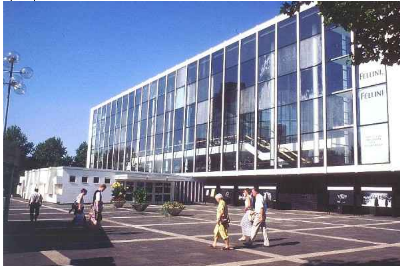
Figure 2.20 Primary Glass Facade
