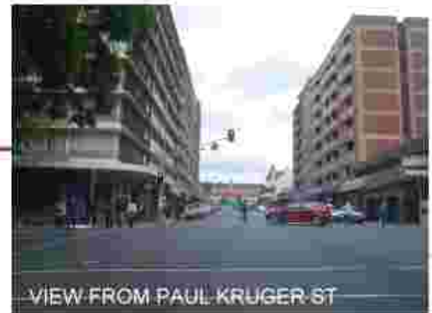
APPROACH TO SITE AND COMMERCIAL
