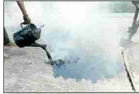
Figure 6.08 Example of roof treatment: Application of Bitumen to roof surface
