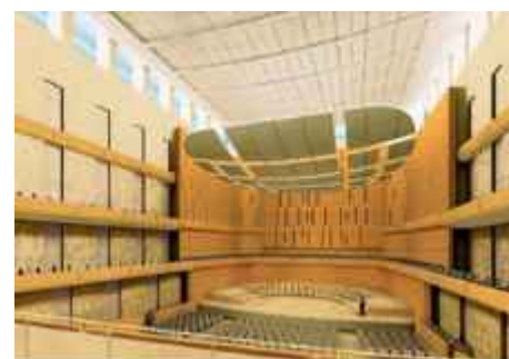
Figure 2.08 Suspended ceiling for acoustic purposes
