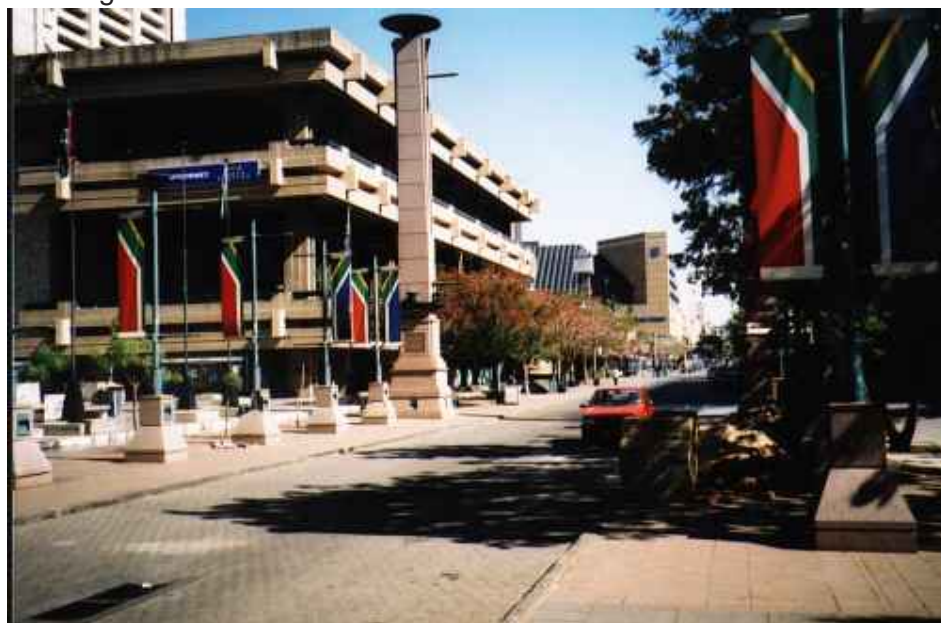
Figure 2.13 Monumental Nature of complex. Relationship with passers by non-existent
