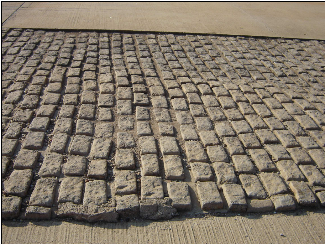
Figure 67: Belgian paving at Gerotek.
