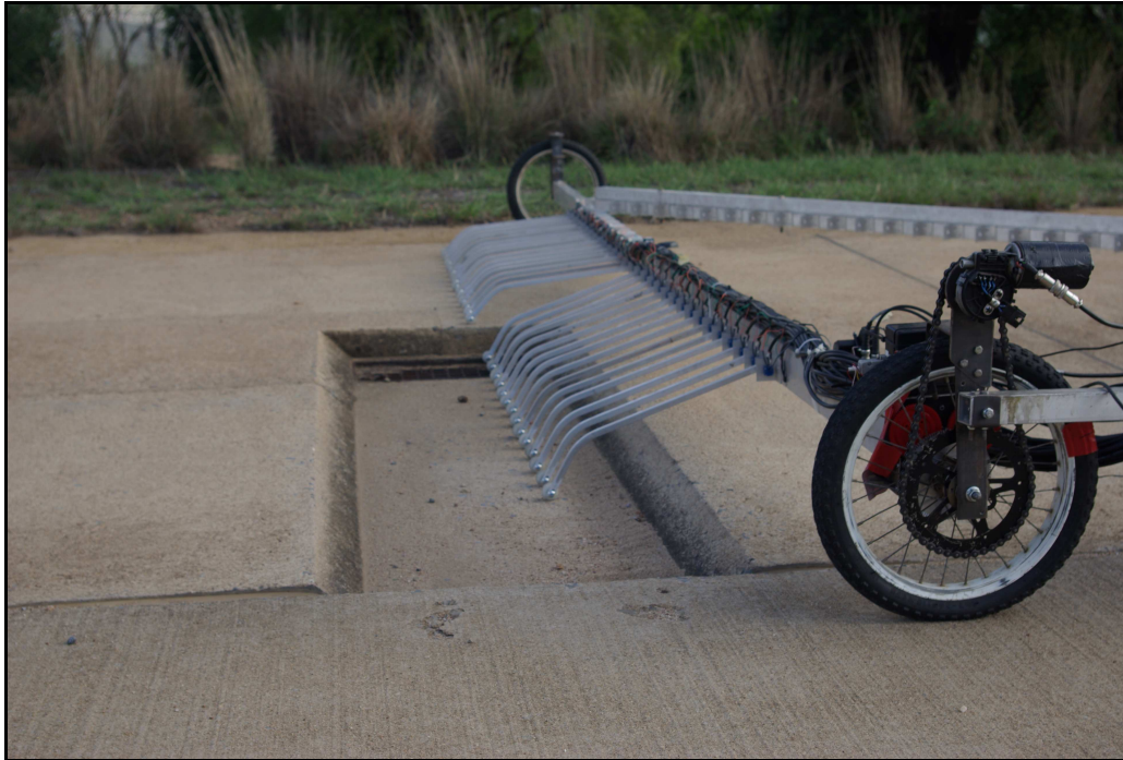
Figure 64: Pothole track at Gerotek.
