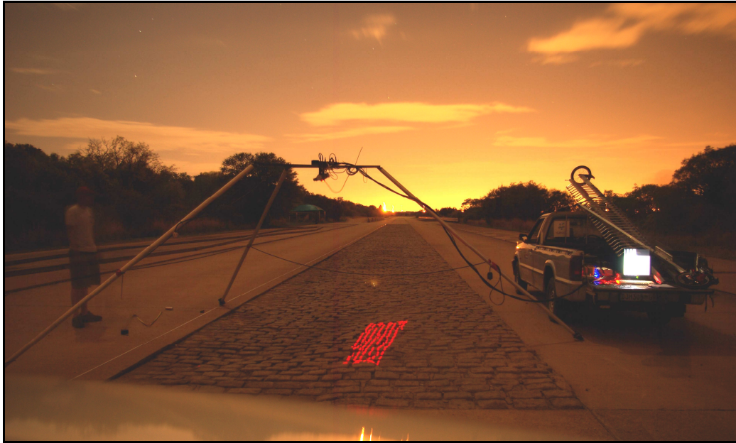
Figure 76: Laser scanner in operation on the Belgian paving at night.
