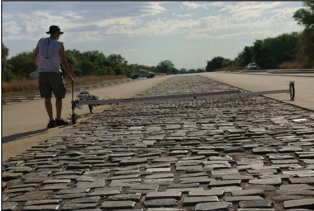
Figure 68: Can-Can Machine profiling Belgian paving.
