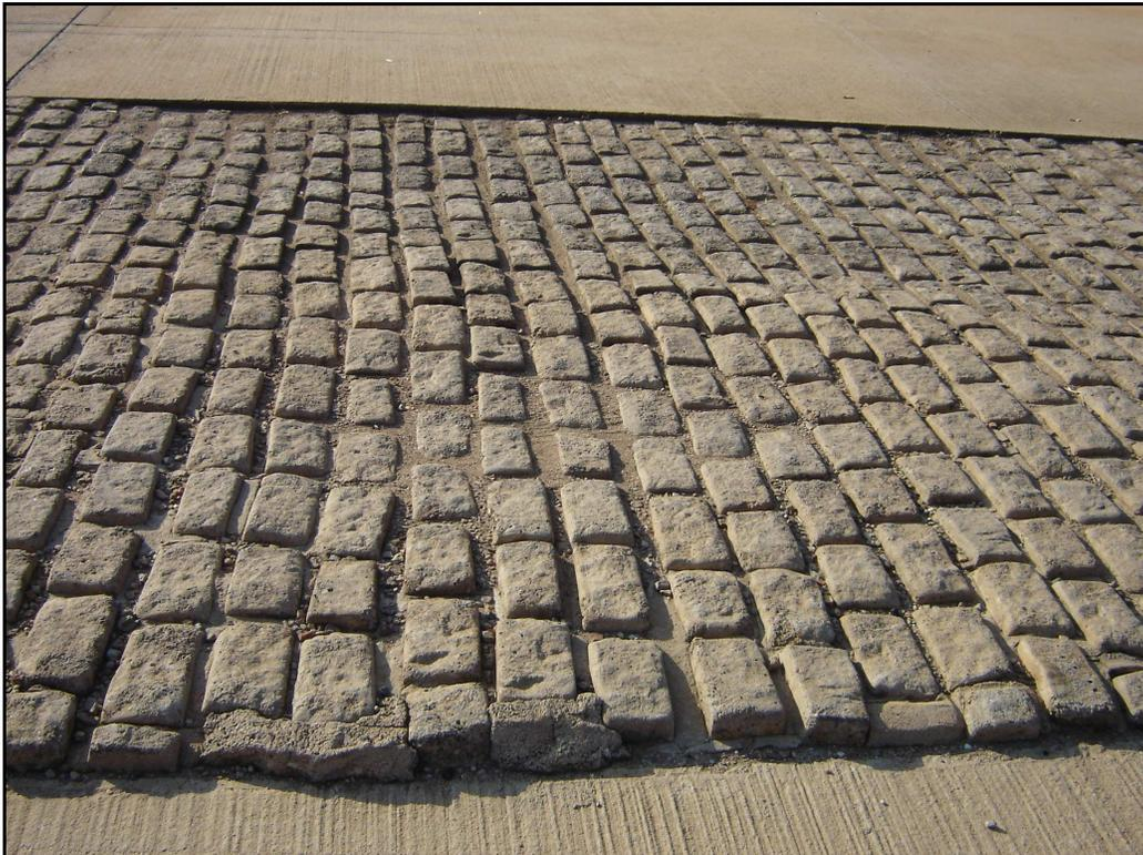
Figure 67: Belgian paving at Gerotek.
