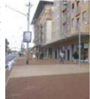
FIGURES 28, 29 28 Public space in 'The Fields' This 'public space' consists of a raised planted platform, removed from the street and from any infrastructure or activity that could stimulate use.
