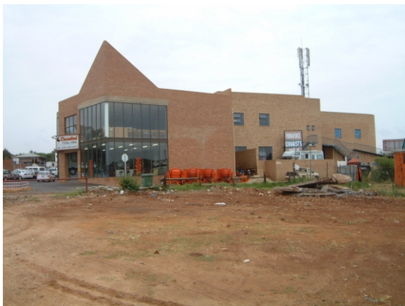
Building on the western side of the HPC.
