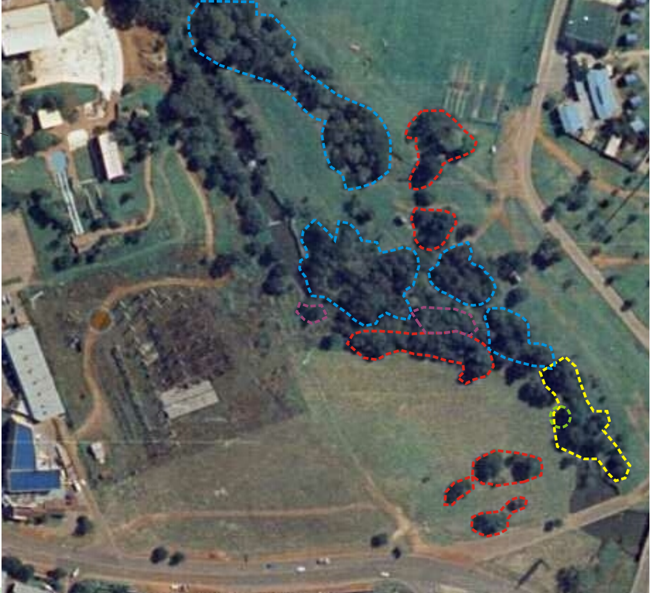
Arial photograph of site
