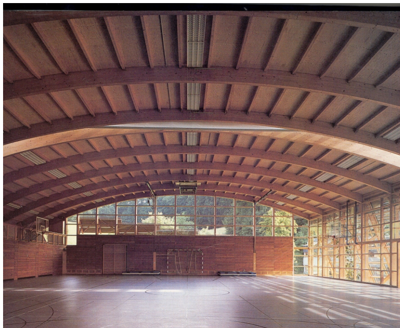
New Sports hall interior
