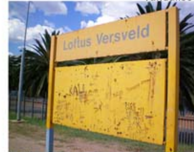
fig. 3.30_Signage on site, vandalised
