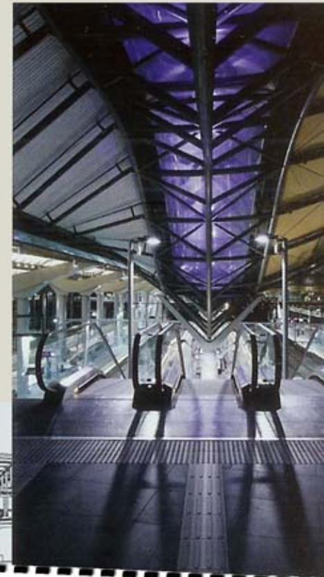
fig. 5.27_ Escalator to platform accentuated by light above
