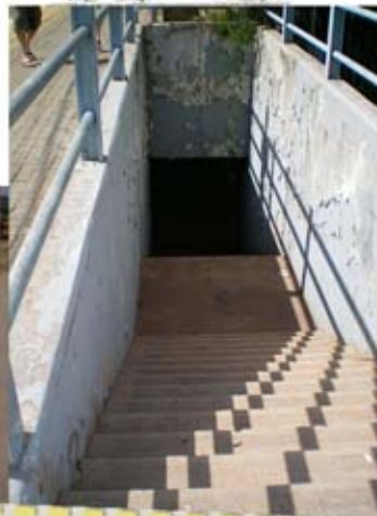
fig. 3.38_ Stairway not in use
