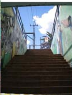
fig. 3.36_ Stairway to platform
