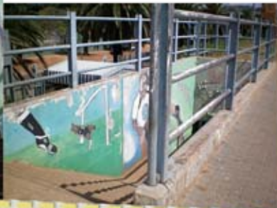
fig. 3.37_ Stairway from platform
