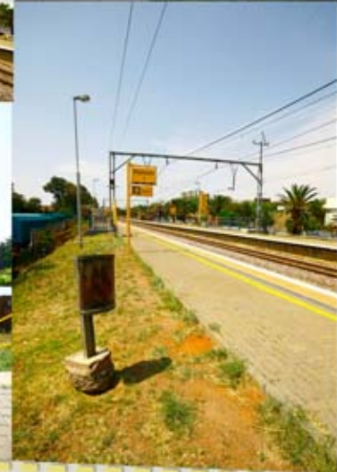
fig. 3.40_ Platform embankment, vandalized litter bin
