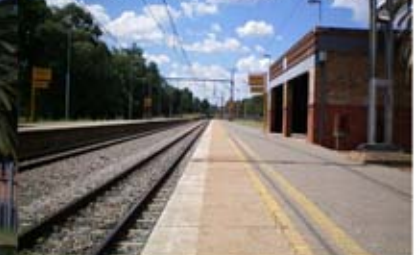
fig. 3.32_Shelter on platform
