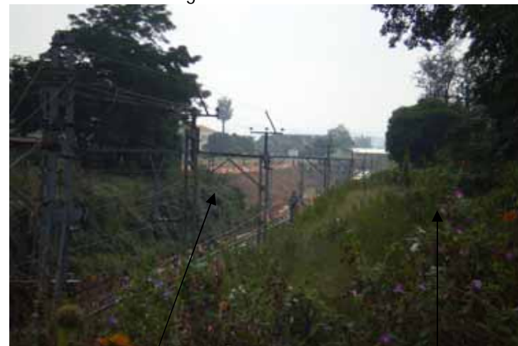
Figure 5: Gautrain Station under Construction
