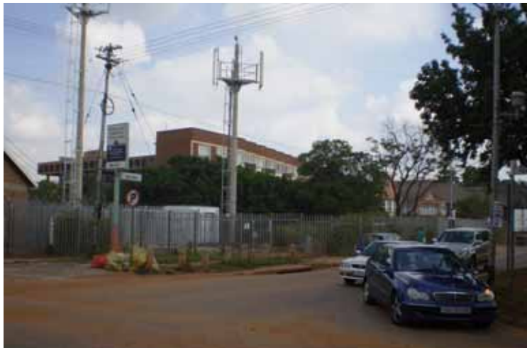
Figure 15: Hilda Street and Park Street junction point
