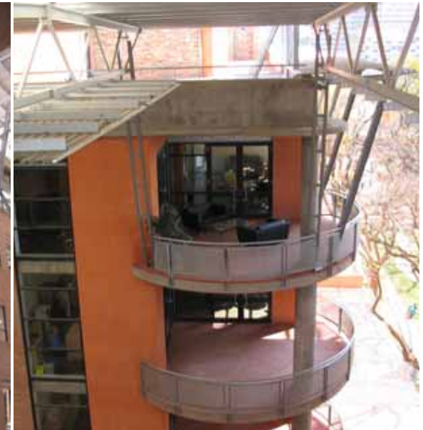
Figure 21: Balconies in the DTI Ref: Korin
