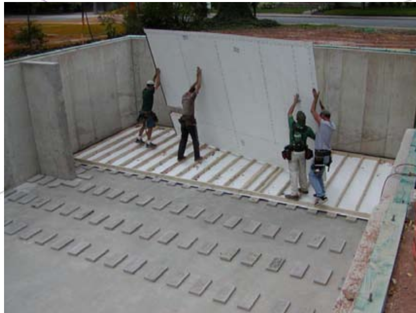
Figure 6.4: Preparation of cavity floor in basement
