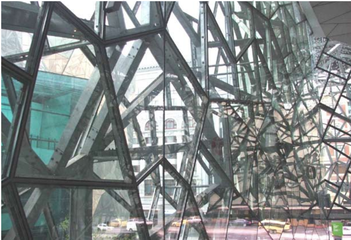
Figure 6.8: Federation Square in Australia, double glazing as part of the fractal facade
