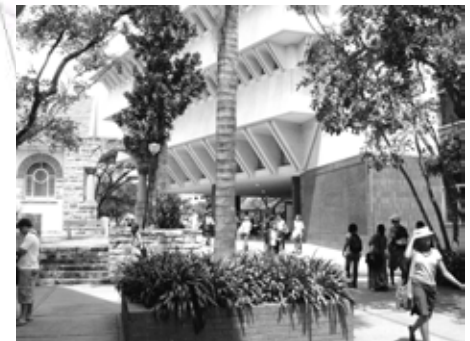
Figure 3.10: Approaching the site under the overhang from the west past the "Kanseliers" Building
