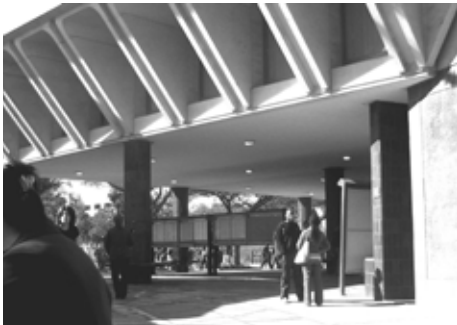
Figure 1.12: Site: Corridor north of existing Library overhang, looking in eastern direction
