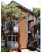
#4 - Marketing Services Building Finished in 1960 (together with "Kanseliers") Function then: Lecturer's Offices Function now: Research Support Offices
