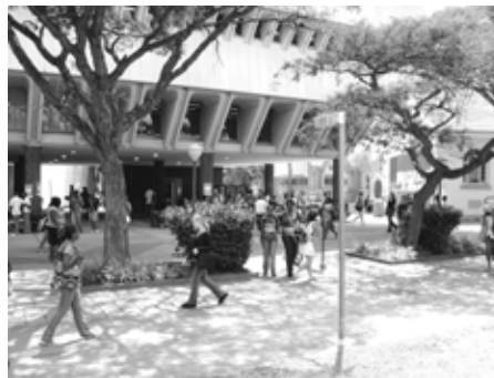
Figure 3.9: Approaching the site under the overhang from the east from the Piazza
