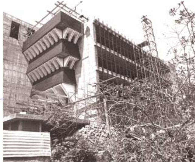
Figure 3.4: Construction of the New Merensky Library
