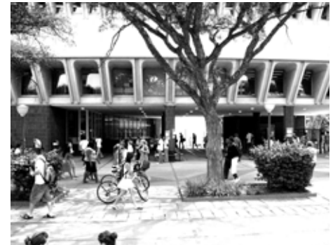
Figure 1.14: Site: Existing Library overhang, looking in western direction
