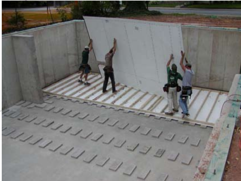
Figure 6.4: Preparation of cavity floor in basement
