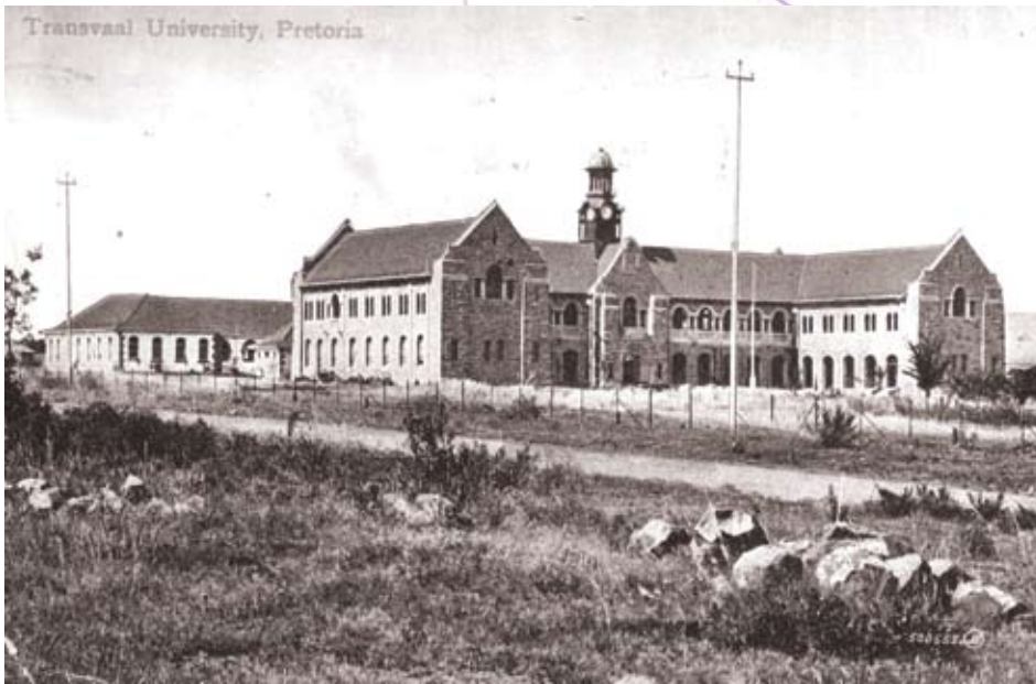
Figure 3.5: The Old Arts building in the foreground with the Old Chemistry building in the background
