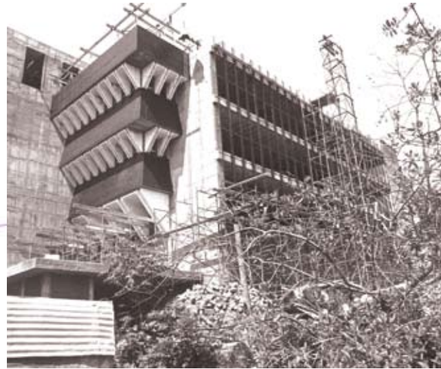
Figure 3.4: Construction of the New Merensky Library
