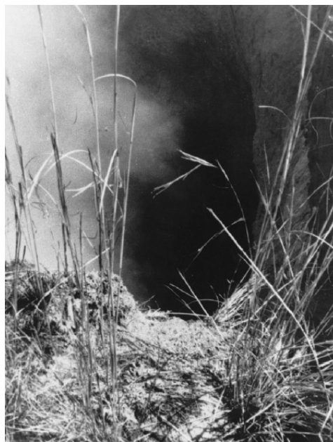
Figure 28. A sulphurous stream emitted from a crownhole (Bell et al. , 2001)
