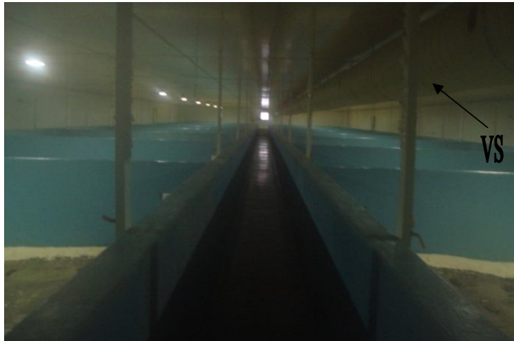
Plate 30: An internal view of the grow house. The columns from the roof carry warm water pipes for the under floor heating. This house is 70m long and contains 2 rows of 9 pens. The vent system (VS) can be seen on the roof which carries fresh (heated) air from outside. A window is present at the back of the house to allow the air pressure to escape.
