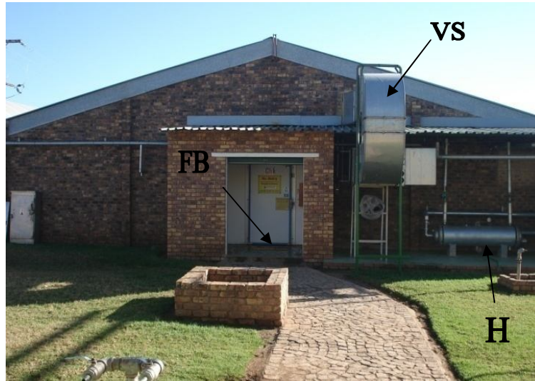
Plate 28: A front view of the grow house, where the vent system (VS) and the water heating system (H) can be seen. This house also has a foot bath (FB) to serve as biosecurity for the crocodiles inside.
