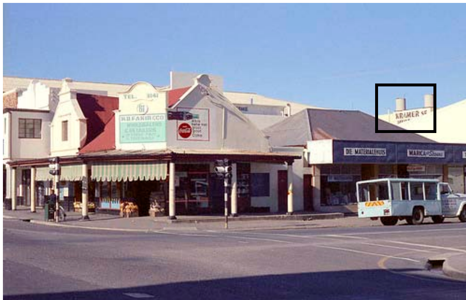
K.B. Fakir & Co, corner of High Street and Stockenström (sic) Street, Worcester, 1972.
