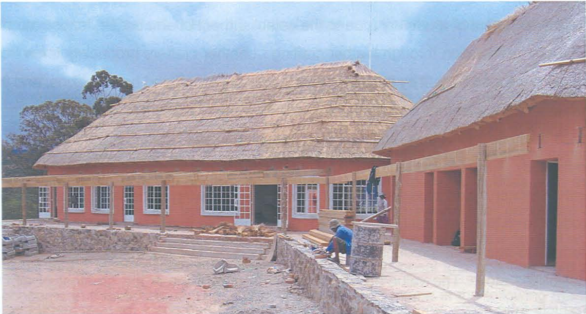
Figure 10.1 Umzimvubu facilities under construction showing the tourist facility nearing completion
