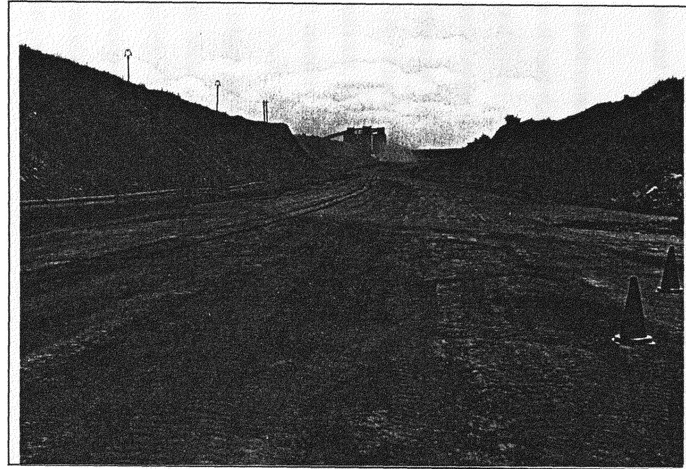
Figure 9.55 Condition of wearing course after blading, Kleinkopje Colliery Site 2.
