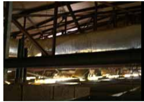
Figure. 129a Structure Lecture halls: roof steel frame
