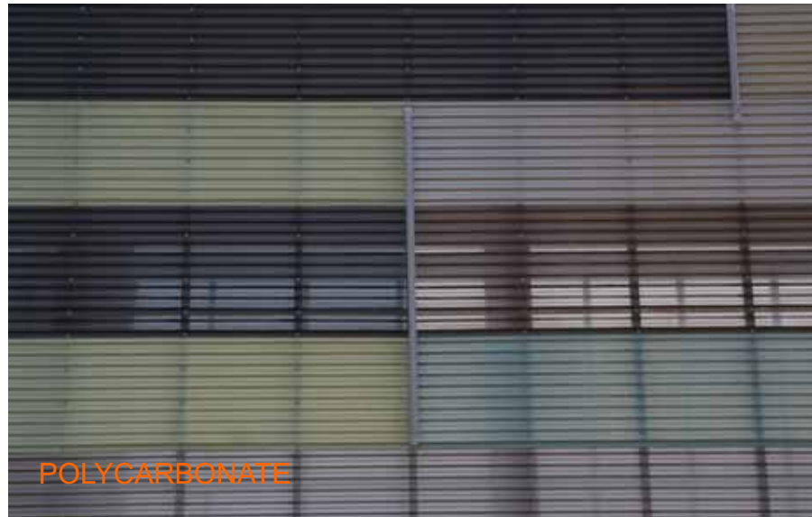
Figure. 124 Materiality: Poly-carbonate sheets Brick work Recycled metal sheets Roof corrugated sheet Concrete panels
