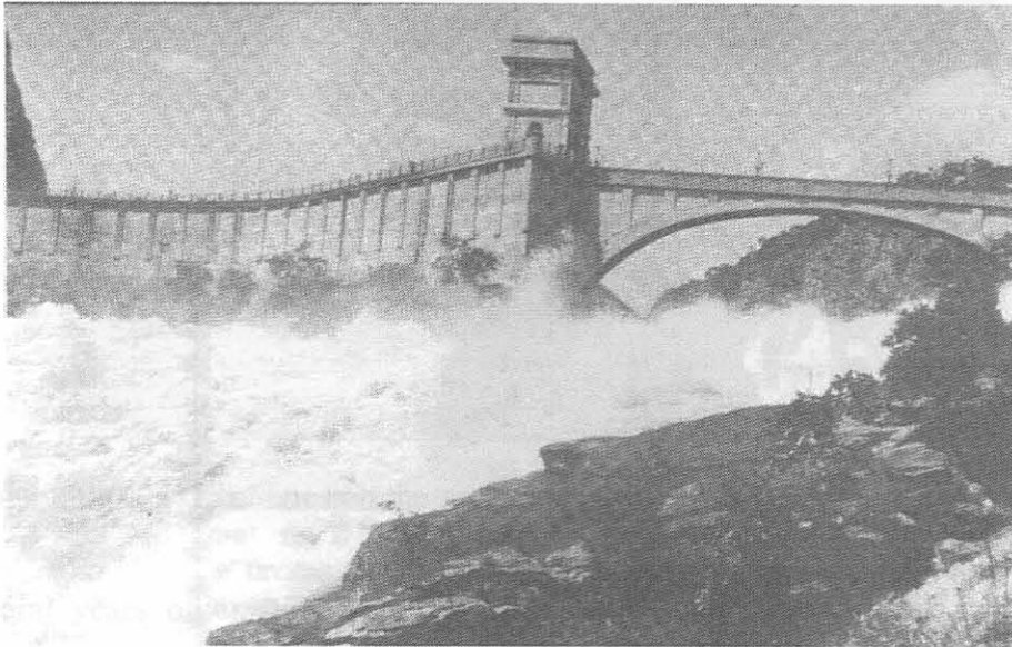
#11 Photograph: (1967) “Hartebeespoort Dam floods”.
