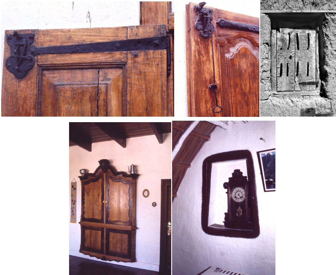
Figure 7.12. Top: Continuity of hinge detail in various Cape vernacular doors (Fagan, 2012b). Bottom: Sophisticated detailing of wall cupboard in Cape Dutch homestead and simple clock niche in vernacular house (Fagan, 2012b).
