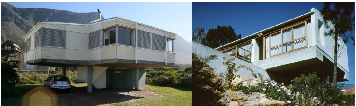
Figure 9.22. Left: House Beyers (1998) showing concrete support system (Author, 2009). Right: Cantilevering supports to House Bertie-Roberts (1965) (Fagan archive - Job No. 644, undated).
