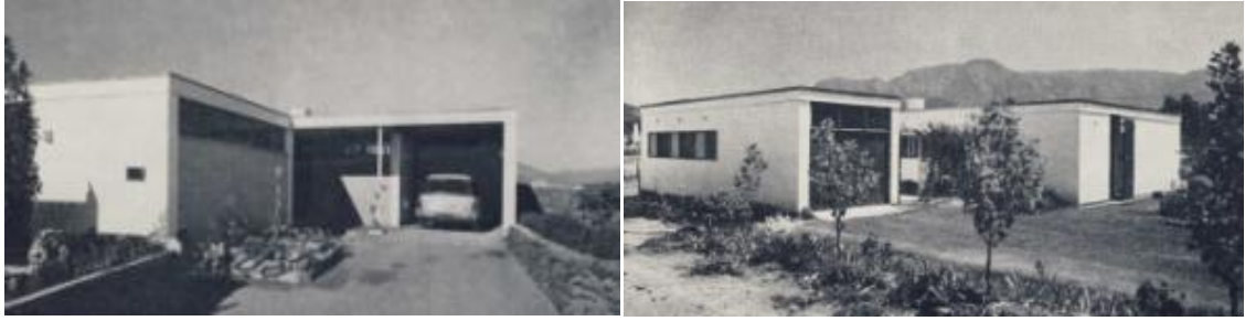
Figure 3.9. Previous page and this page left: Plan of and garden and entrance views to House Ross, Worcester, Western Cape (1955) (Fox, 1998:83) and Architect and Builder, April, 1958:46). Previous page and this page right: Plan of and garden and entrance views to House Fox, Worcester, Western Cape (1955) (Architect and Builder, April, 1958:42-45).
