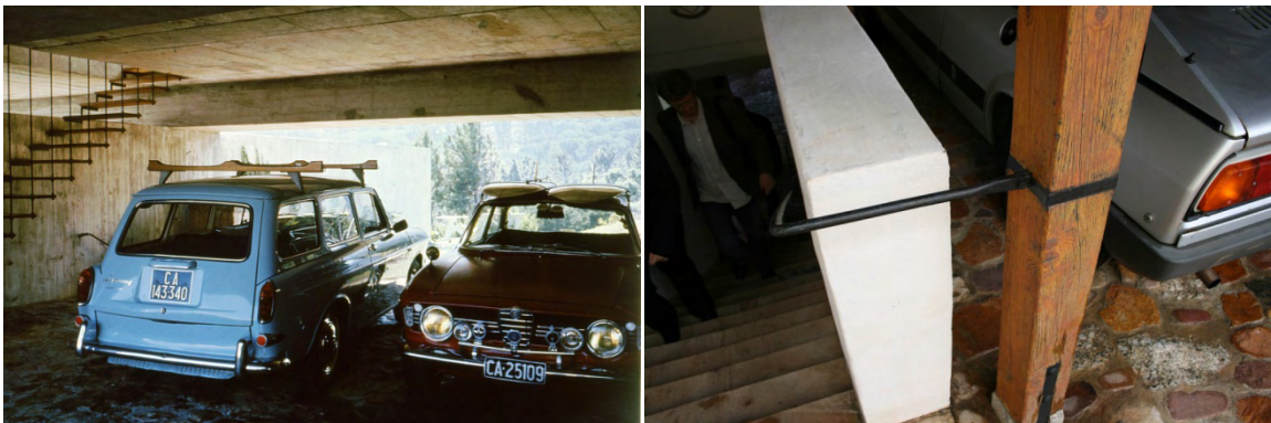
Figure 10.31. Left: House Bertie-Roberts entrance stair from carport (Fagan archive - Job No. 644, undated). Right: Entrance wall, carport column and steel rod handrail leading to front door (Author, 2009).
