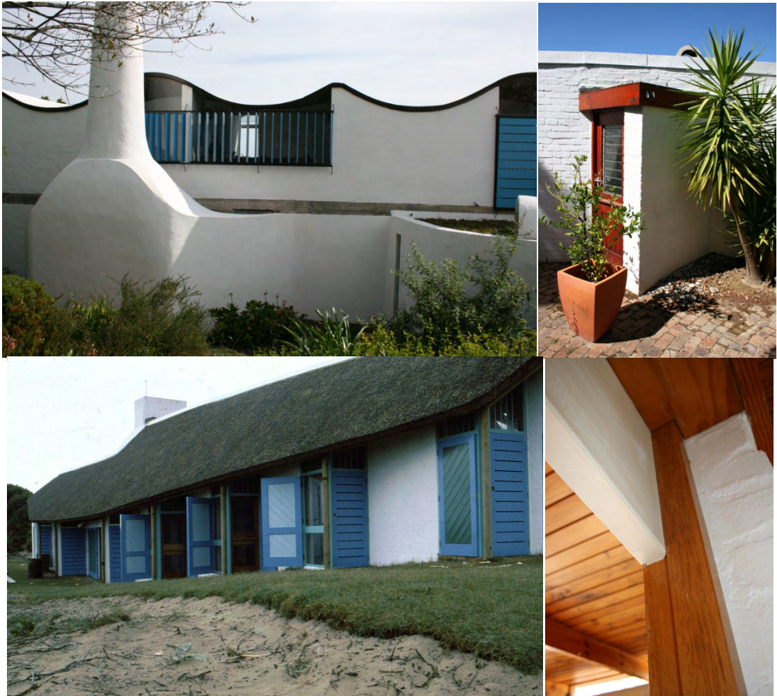
Figure 10.26. Top Left: Exposed first floor concrete floor slab to House Die Es (1965) (Author, 2008). Top right: Bagged and painted brickwork to House Blommaert (1982) (Author, 2009). Bottom left: Differing internal and external colours to doors at House Swanepoel in Cape St. Francis (1980) (Fagan archive - Job. No. 8011, slide collection IC, undated). Bottom right: Bagged and painted brickwork and timber beams and ceilings to House Blommaert (1982) (Author, 2009).
