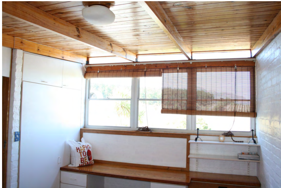
Figure 7.3. Previous page left: Glazed fanlight to passageway at House Levin (1969) (Author, 2009). Previous page middle: Frameless top glazing to door at House Raynham (1967) (Author, 2008). Previous page right: 'Frameless glazing' to western edge of living room to House Patterson (Author, 2008). Above: Glazing between roof rafters to House Blommaert (1982) (Author, 2009).
