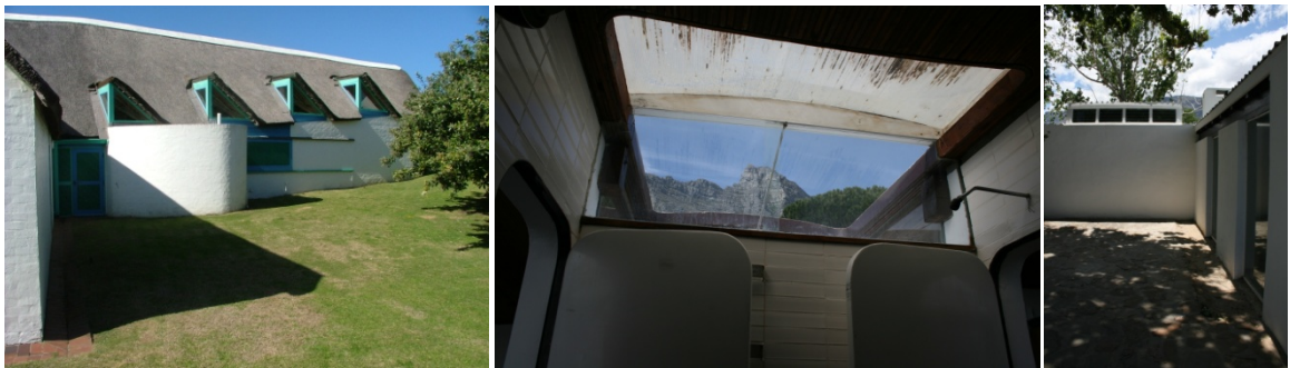
Figure 9.21. Left: Moulded rooflights to House Swanepoel in Cape. St. Francis (1980) (Author, 2005) . Middle: View through rooflight to bathroom of Die Es (1965) (Author, 2009). Right: Raised rooflight to House Wolfaardt (1965) (Author, 2009).
