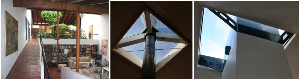
Figure 7.7. Left: Foyer and dining area of House Keurbos (1951) flooded with light from glazed roof over (Author, 2008). Middle and right: Steel roof collars to House Beyers (1998) and House Swanepoel in Hermanus (1990) act as roof and flue supports (Author, 2009).
