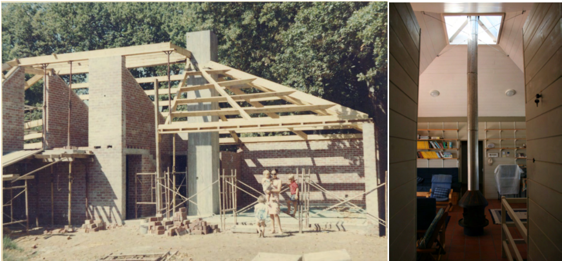
Figure 10.7. Left: Fireplace flue as roof support to House Raynham (1967) (Photo courtesy of the Raynham's, 2009). Right: Fireplace at House Beyers (1998) (Author, 2009).
