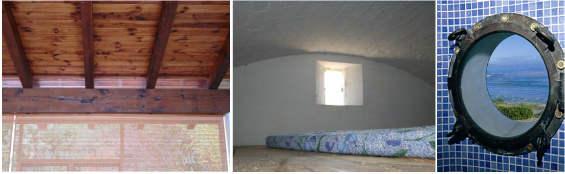
Figure 10.29. Left: Sliding glazed panels between rafters at House Keurbos (1951) (Author, 2008). Middle: Window to mezzanine over passage at House Paradys (2003) (Author, 2009). Right: Porthole at House Paradys (2003) sea facing bathrooms (Fagan, 2012b).
