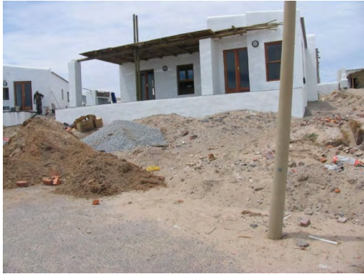
(Photograph of house under construction (Fagan archive, undated).
