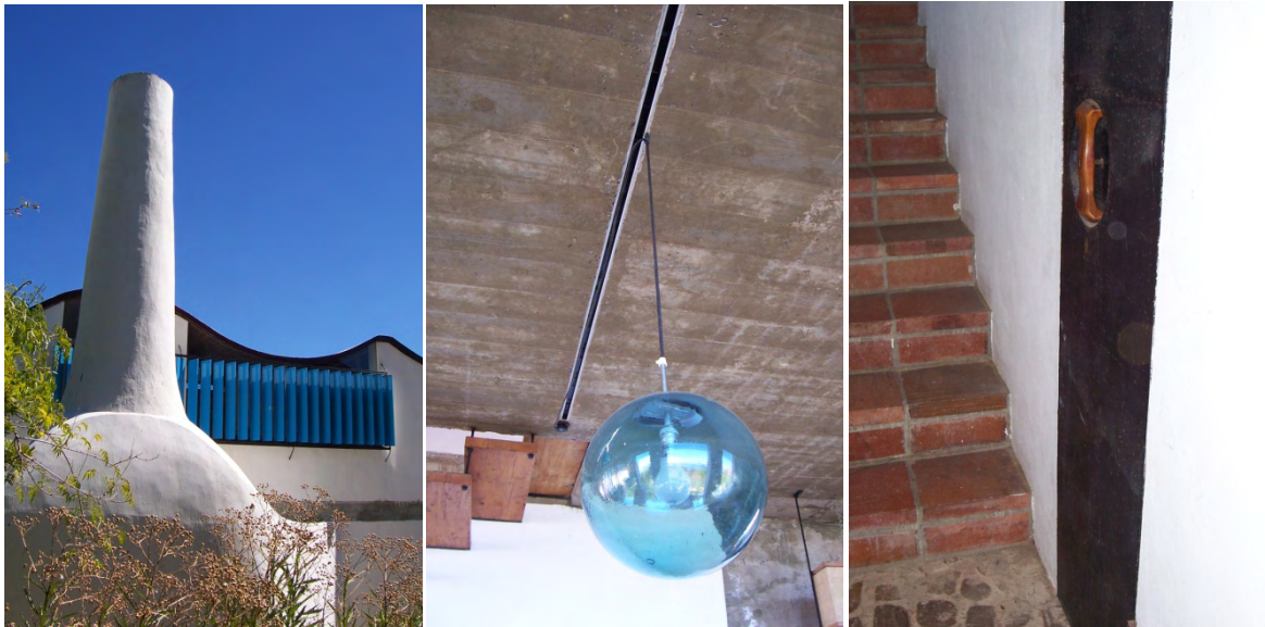
Figure 7.41. Die Es (1965): Chimney; in-situ concrete first floor, timber treads and Japanese fishing buoy as lamp; quarry tile stairs leading to basement (Photo's courtesy of Auret, 2006).
