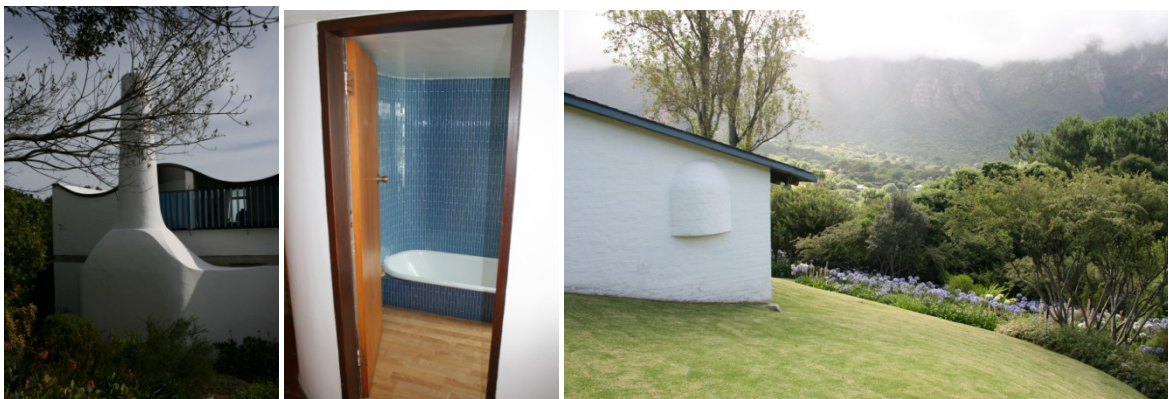
Figure 9.5. Left: House Die Es (1965) organically shaped chimney (Author, 2009). Middle: Curved wall of lower ground floor bathroom to House Keurbos (1951) (Author, 2009). Right: Niche to living room of House Keurbos (Author, 2009).
