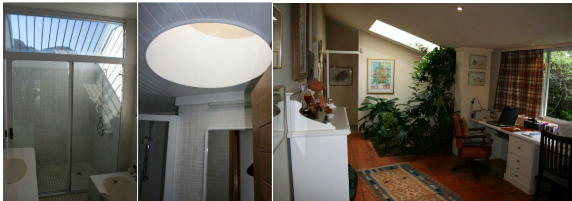
Figure 10.9. Left: Main bathroom courtyard at House Swanepoel in Hermanus (1990) (Author, 2009). Middle: Bathroom rooflight at House Swanepoel in Hermanus (1990) (Author, 2009). Right: Rooflight over small internal garden to House Auldearn (1992) (Author, 2008).
