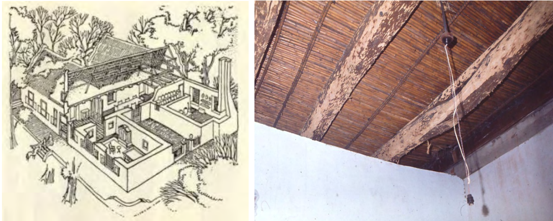
Figure 7.8. Left: Biermann's sketch (to which Fagan often refers) showing the spatial and constructional layout of the traditional Cape house (Biermann, 1995:37). Right: Timber tie beams of roof truss supporting floor of roof space (Fagan, 2012b).
