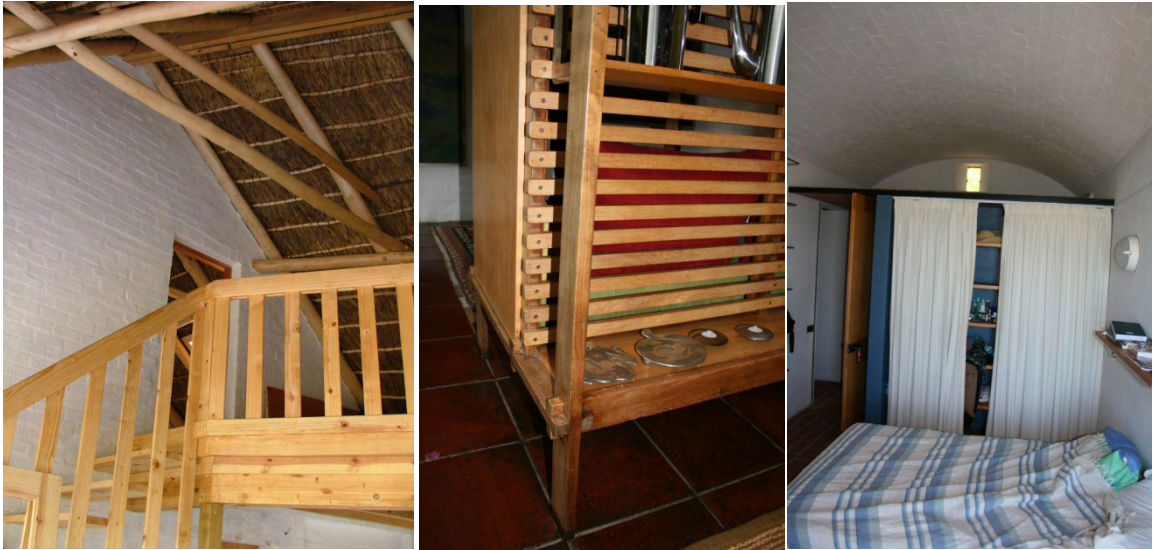
Figure 10.17. Top left: Balustrade as screen wall in House Fagan in McGregor (2005) (Author, 2009). Middle: Cupboard as screen between hall and dining area of House Keurbos (1951) (Author, 2008). Top right: Curtained cupboard to bedroom of House Paradys (2003) (Author, 2009).
