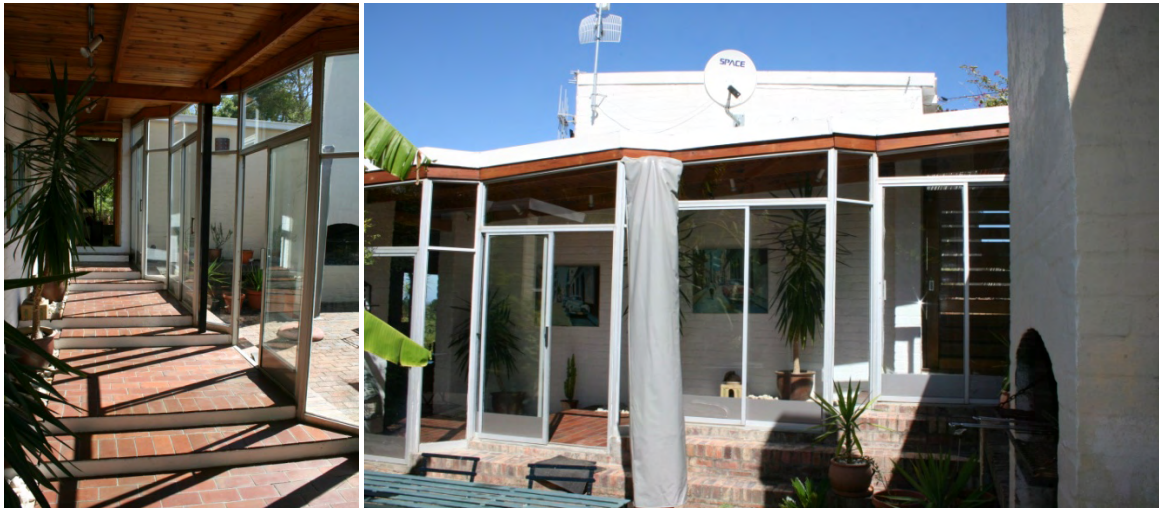
Figure 10.12. Left: Glazed walkway to bedrooms at House Blommaert (1982) (Author, 2009). Right: View from courtyard to glazed walkway at House Blommaert (1982) (Author, 2009).
