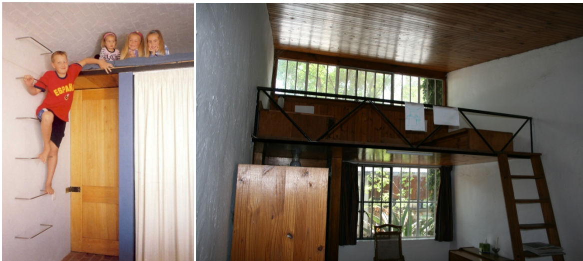
Figure 9.18. Previous page left: Playroom of House Raynham (1967) (Author, 2008). Previous page right: Loft space over passage to House Swanepoel in Cape. St. Francis (1980) (Fagan archive - Job No. 8011, undated). Left: Loft space over passage to House Paradys (2003) (Fagan archive - Job No. 0205, undated). Right: Loft space in bedroom of Hellmut Stauch's House Hakahana (1951) (Author, 2008).
