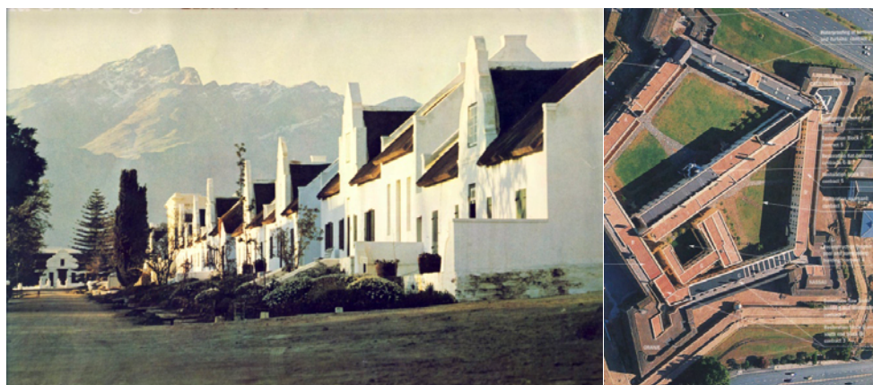
Figure 7.40. Left: Main Street of Tulbagh restored by Fagan after the earthquakes of 1969 (Fagan, 1975:cover). Right: Aerial view of the Castle restored by Fagan from 1969 to 2002 (Anon, 2002:43).
