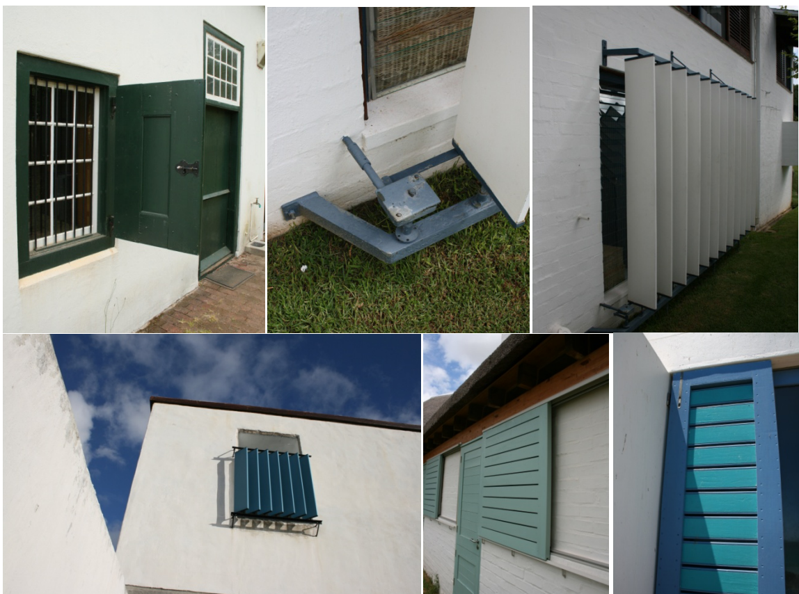
Figure 9.20. Top left: Shutter to Non Pareille homestead, Paarl (1876) (Author, 2007). Top middle and right: Shutter opening mechanism and shutter to House Keurbos (1951) (Author, 2008). Bottom left: Shutter to main bedroom at Die Es (1965) (Author, 2008). Bottom middle: Sliding shutter to House Fagan in McGregor (Author, 2009). Bottom right: Hinged and ventilated shutter to House Paradys (2003) (Author, 2009).
