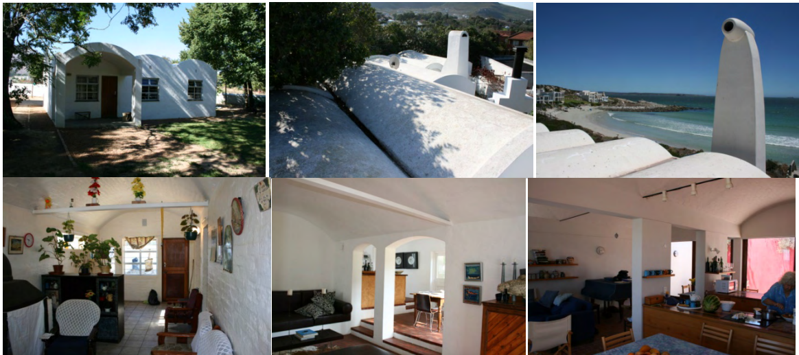
Figure 10.14. Top and bottom left: Exterior and interior views of barrel vaulted roofs at Houses at Idas Valley (1975) (Author, 2008). Middle: Exterior and interior views of barrel vaulted roofs at House Blommaert (1982). Right: Exterior and interior views of barrel vaulted roofs at House at House Paradys (2003) (Author, 2009).
