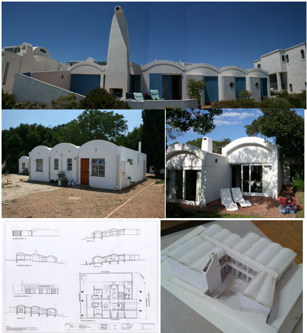
Figure 7.11. Top: Barrel vaulted roof at House Paradys (2003) (Author, 2009). Middle left: Barrel vaulted roofs to Idas Valley (1975) (Author, 2009). Middle right: House Lückhoff (1981) (Author, 2009). Bottom left: Proposed house with barrel vaults and linking mono pitch roofs to House Van Zyl (2007) (Fagan archive - Job No. 0702 24/03/2006). Bottom right: Model of House Visser (Author, 2012).
