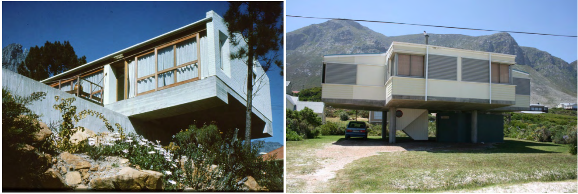
Figure 7.27. Previous page left: Plan of House Bertie Roberts (1965) (Anon, 1968:12). Previous page right: Ground plan of House Beyers (1998) (Fagan archive - Job No. 9813. Left: Concrete service beams at House Bertie-Roberts (1965) (Fagan archive - Job No. 644,undated). Right: Concrete columns and cantilevered beams and slab at House Beyers (1998) (Author, 2008).
