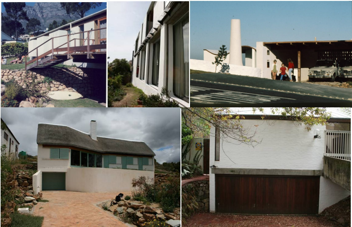
Figure 9.8. Top left: Stone retaining wall at House Bertie-Roberts, Camps Bay (1966) (Fagan archive - Job No. 644, undated). Top middle: House Die Es (1965) showing junction with ground (Author, 2009). Top right: Die Es, Camps Bay, (1965) still under construction (Fagan archive - Job No. 656, undated). Bottom left: House J.J. Fagan, McGregor (2005) (Author, 2008). Bottom right: House Raynham, Newlands (1967) (Author, 2008).
